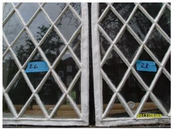
but this is a fundamentally flawed approach. The lead would accelerate the corrosion of the iron, and thereby the deterioration of the windows. The hinges and pins, and screws are also corroded and falling out.
