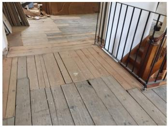
2.1.5. The boards in the rear room run parallel to the rear elevation across the building. The joists below this run across the rear room from back to front. There is a modern boarded area over the utility room consistent with the location of a spiral staircase on the 1973 drawing. This is consistent with the removal of a stair indicated in the drawing. The direction of the boards indicates that the joists within the utility room run in the
