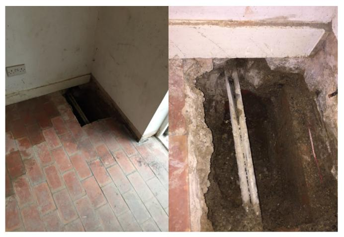
protection or insulation. The pipework, and the slab, appears to run below the internal wall, with the slab thicker at the wall position.
