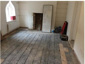
long direction. This is consistent with the wall below not being an original supporting wall for joists in the narrow direction. The evidence is consistent with the 1972 drawings which indicate a wall removed at first floor level and the floor being reconstructed at this location.
