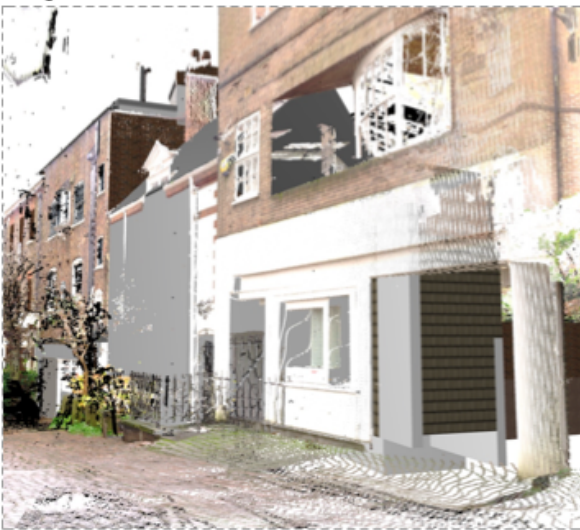
Existing Far view
