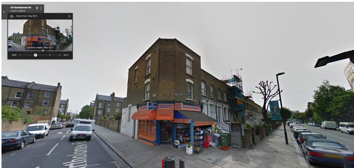
Picture above - May 2012
