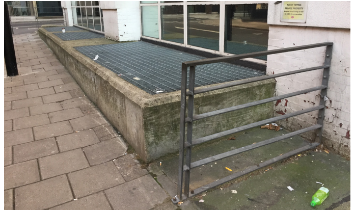
Balustrade and upstand adjacent to Tottenham Street Entrance
