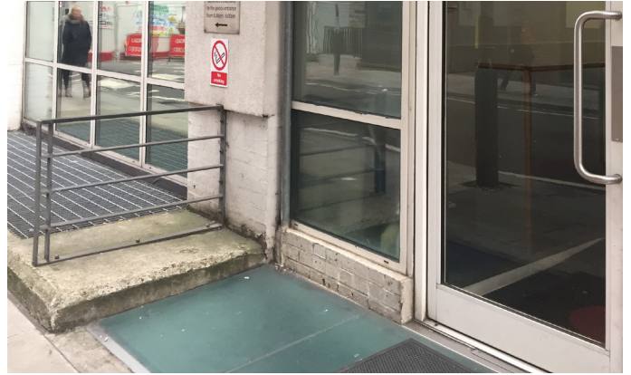
Balustrade and upstand adjacent to Cleveland Street Entrance
