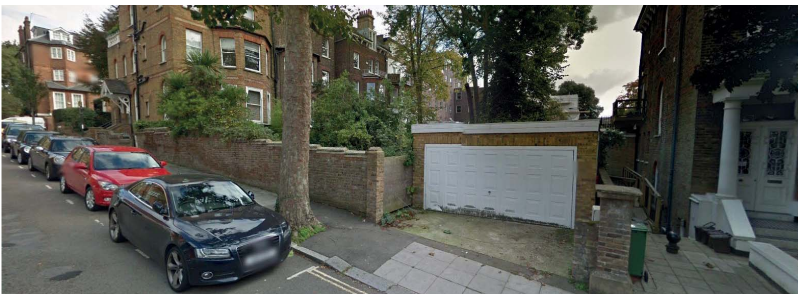
Current appearance (view from Ellerdale Road)
