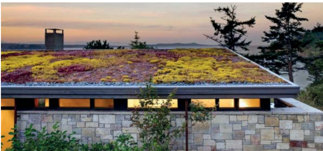
Examples of green roof
