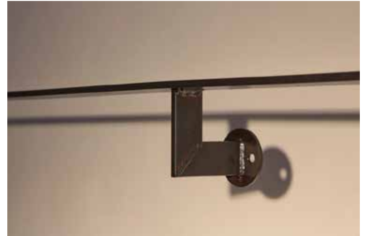
handrail, black painted steel
