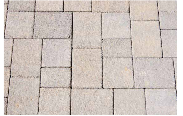
permeable interlocking paving
