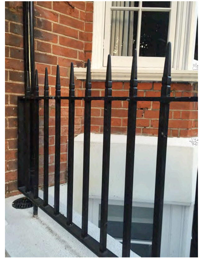
Existing Railing at Neighbouring 34 Ferncroft Ave
