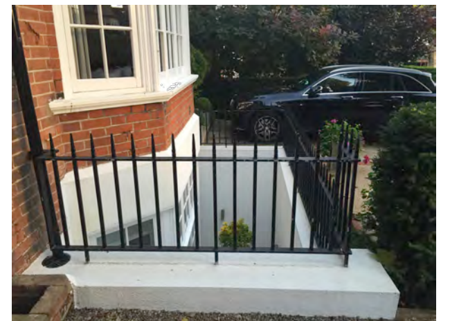
Existing Railing at Neighbouring 34 Ferncroft Ave
