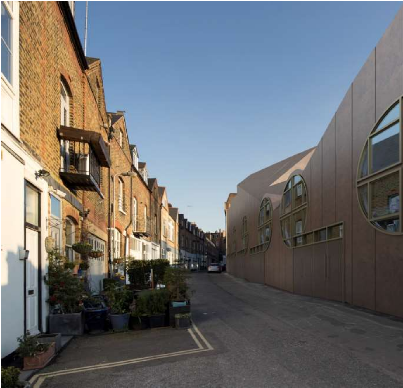
Figure B2: Proposed development site view from Canfield Place looking east. The noise sensitive receptors are on the left hand side of the road and the development site is on the right hand side.
