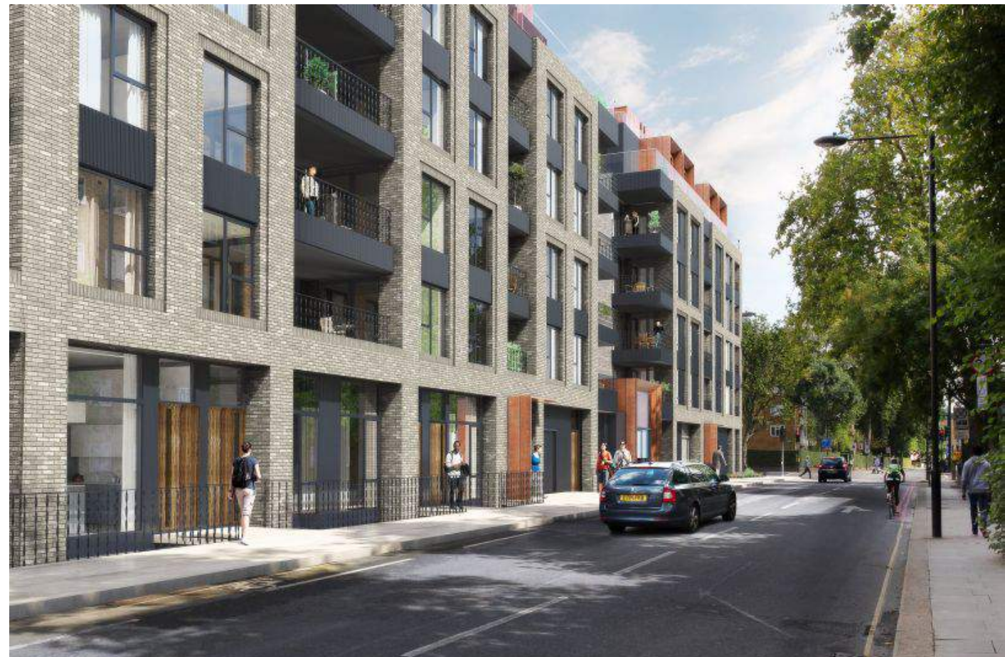
This development currently in construction is situated 2 mins walk away from our proposed x5 houses, x1 Flat and Gallery space development on Rochester Square
