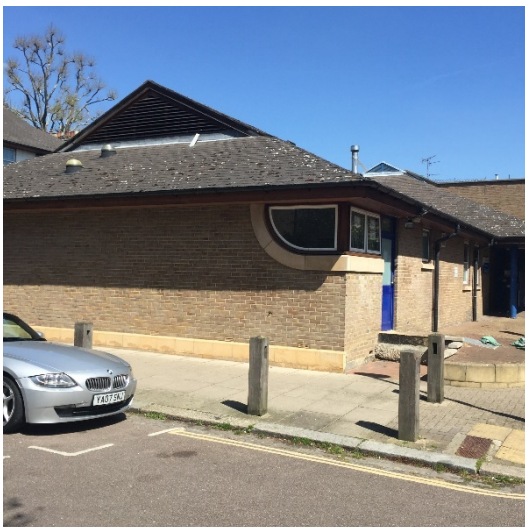
Pic 1 – NHS Community Recovery Building
