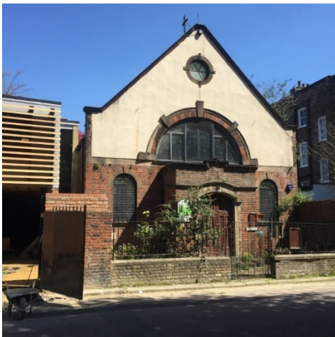
Pic 5 – Existing Building from the South
