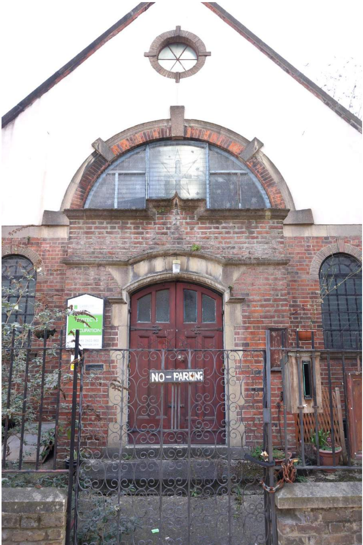
Detail of the street front and main entrance
