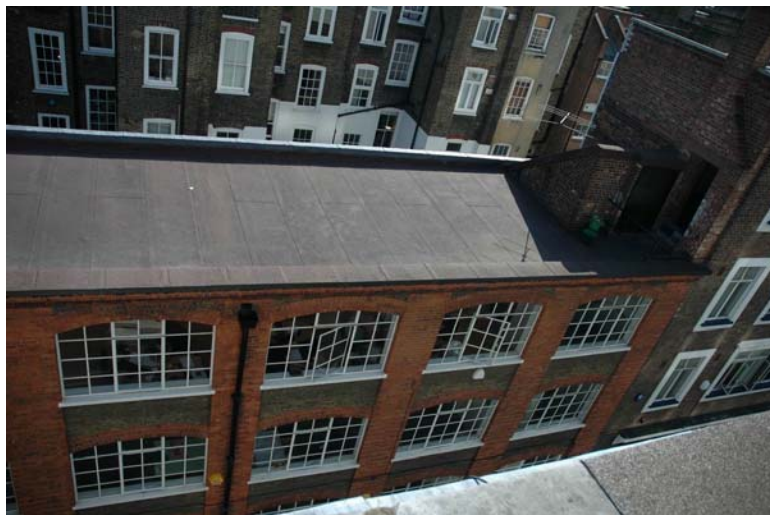
Photograph 3. 14-18 Emerald Street Roof / Staircase enclosure
