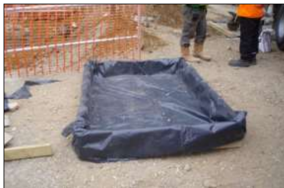
Pollution image 2: Soil bunding or a supporting framework covered in heavy-duty plastic sheeting is essential where there is a risk of spillages contaminating RPAs. This specifically applies to cement mixing areas and vehicle washing facilities.
