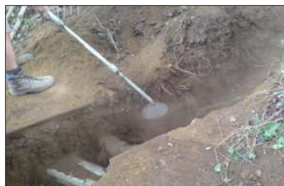
Excavation image 2: Air spades are very effective at exposing
