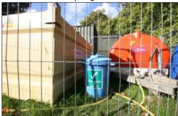
Pollution image 1: Where fuel or other chemicals are stored on site, it is now standard practice to have emergency spillage kits available to restrict the environmental impact of accidents.
