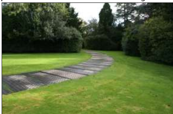
Hard surfacing/structure removal image 1: Ground protection must be used where repeated foot or vehicle traffic could cause compaction in sensitive RPAs. It can be as simple as plywood for pedestrians, but must be more robust for vehicles.
