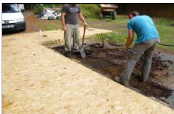
Excavation image 1: Careful hand-digging using conventional
