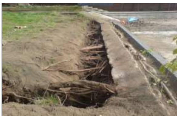
Excavation image 3: Air spades are particularly useful where roots are very dense.
