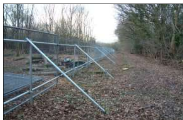
Fencing image 2: Heras fencing wired to scaffold braced posts is a robust and effective interpretation of the BS specification.
