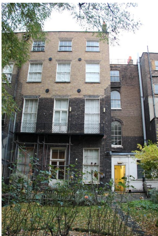
1 Montague Street - Rear Elevation
