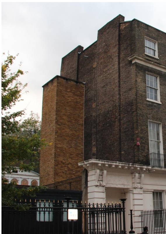
1A Montague Street - Side elevation Existing lift shaft. Existing boiler flue to be removed.
