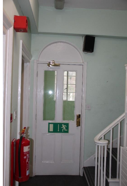
Existing window to undergo full overhaul to ensure good working condition and receive full redecoration. Existing door to access stairs to first floor to be removed. Main stone stair to be redecorated.
