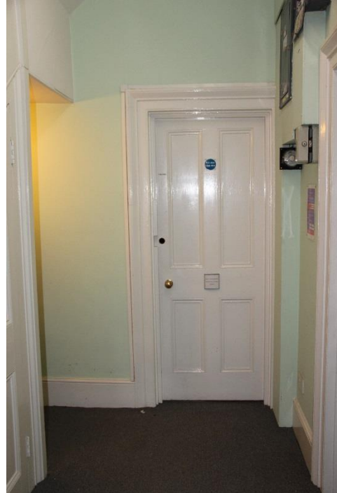
Existing door openings to be infilled where necessary and finished to match adjoining walls
