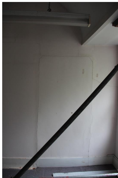
New opening to be created within timber stud wall. Refer to detail drawings (70)AD031/032 and structural engineers information;
