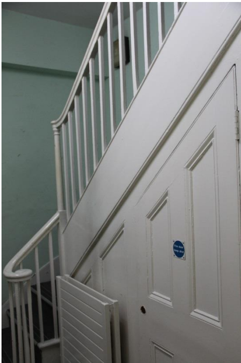
Timber stair and associated panelling to be redecorated. Existing door linking 1MS to be upgraded to a 30min fire protected door. Panels adjacent to the door should be over clad on the fire side (non-stair side) with a fire resistant board that achieves 30 minutes fire protection.
