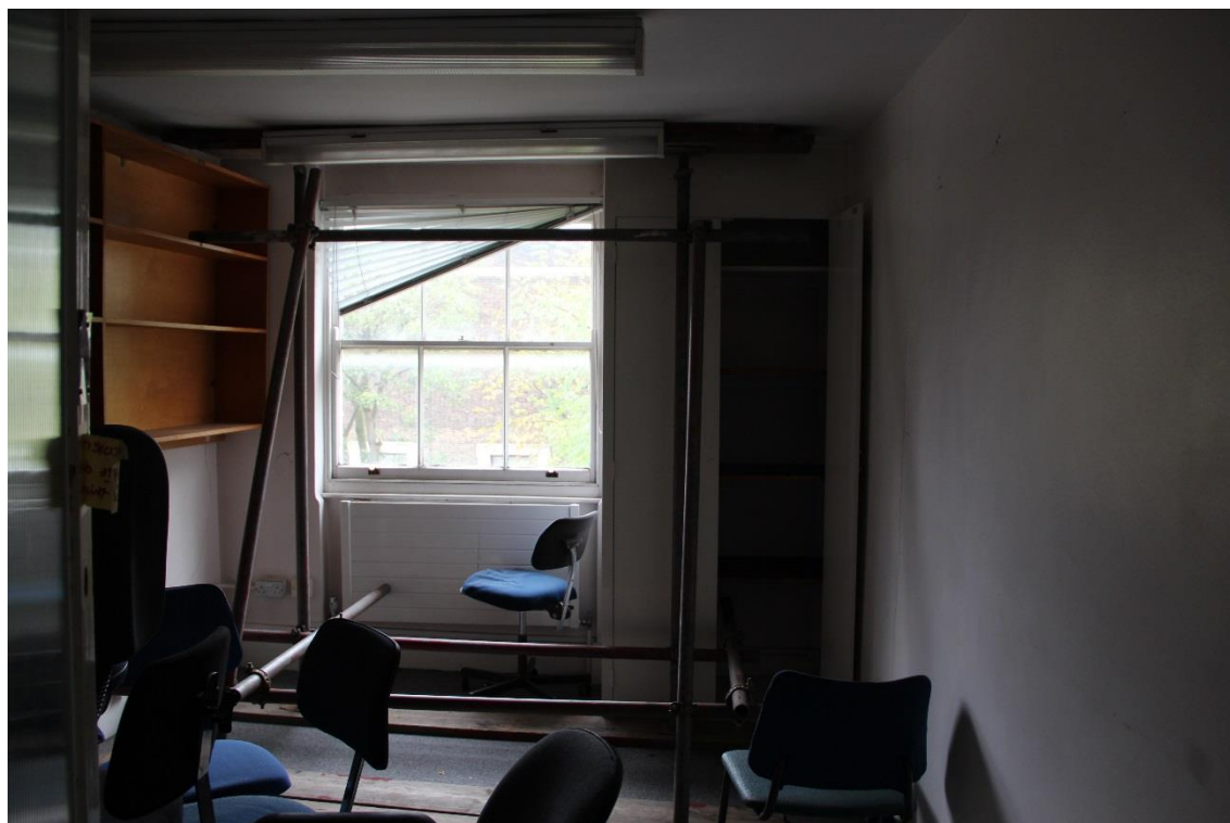
Existing room 1MS/5/013:
