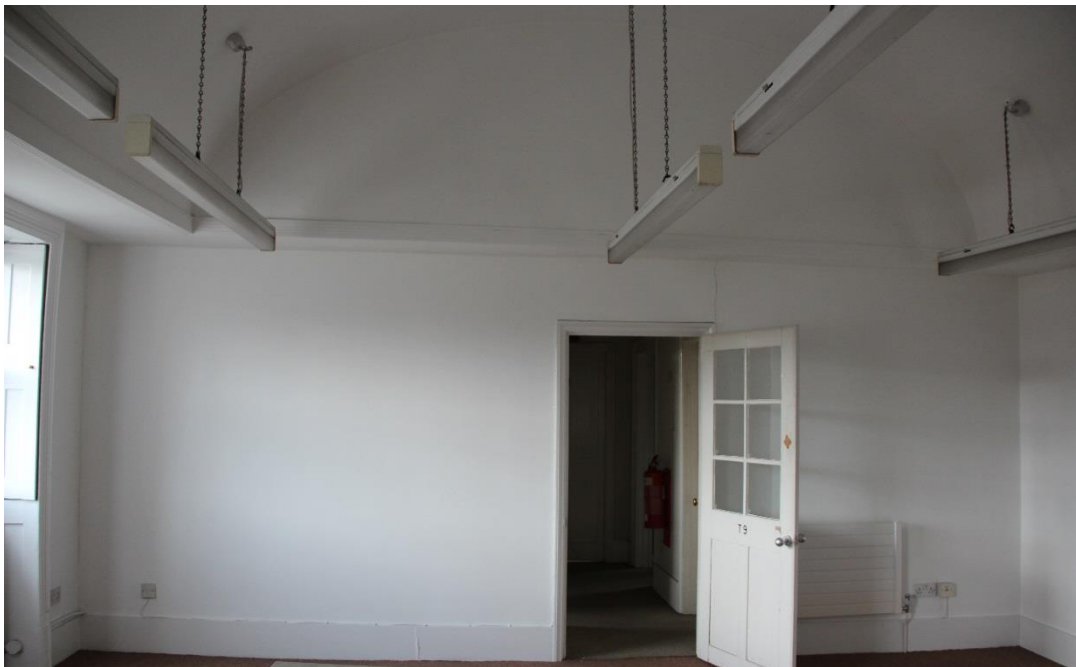
Existing door to be removed and opening to be infilled. Finish to match adjoining walls
