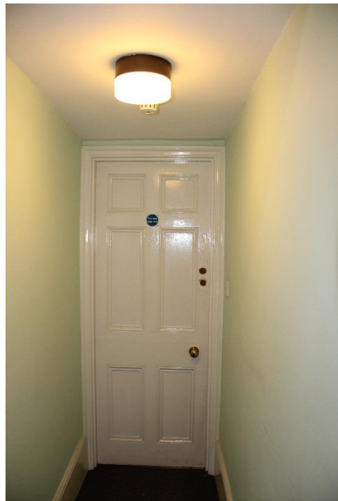
Timber stair and associated panelling to be redecorated. Existing door linking 1MS to be upgraded to a 30min fire protected door. Panels adjacent to the door should be over clad on the fire side (non-stair side) with a fire resistant board that achieves 30 minutes fire protection.
