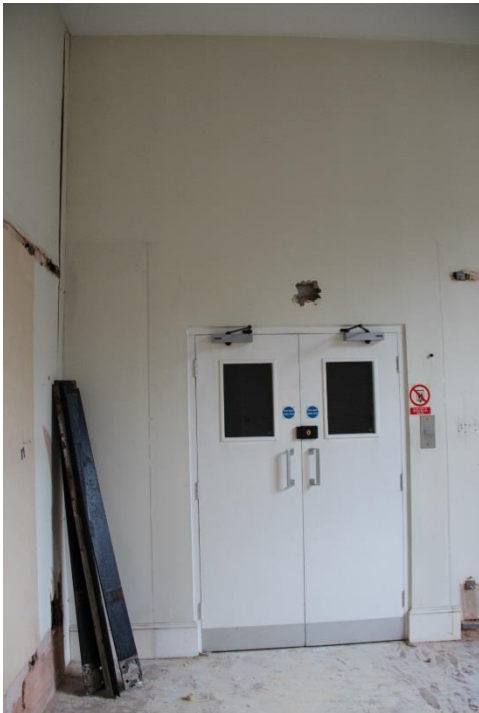
ELEVATION 3 - Metal work and damaged modern plaster finishes to be carefully removed and replaced with original plaster to match existing adjacent. Redecoration throughout. New FD30 double doors to replace existing lift shaft doors to match design of adjacent doors. Refer to detail drawing (32)AD002
