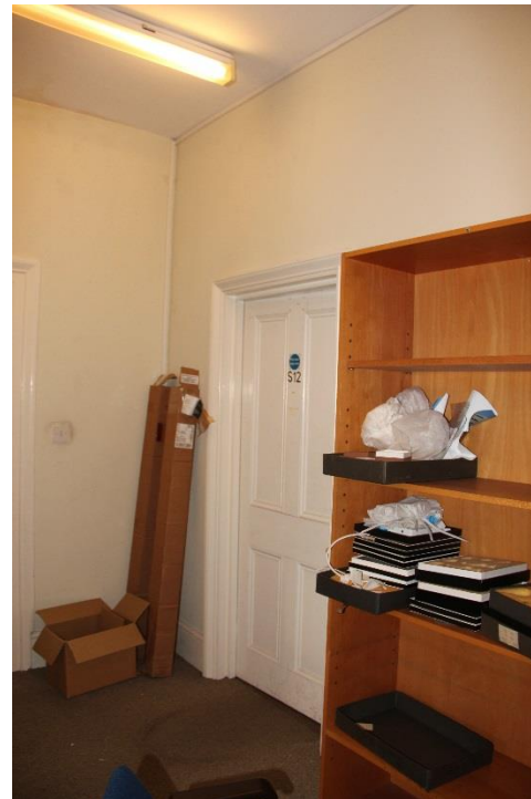
Existing room 1AMS/4/014: Existing door to be retained and redecorated; Wall adjoining room 1AMS/4/012 to be completely removed. Adjoining walls to be made good where necessary. Redecoration throughout.
