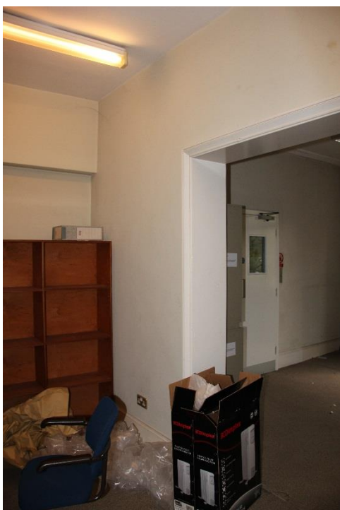
Existing room 1AMS/4/014: Existing door to be retained and redecorated; Wall adjoining room 1AMS/4/012 to be completely removed. Adjoining walls to be made good where necessary. Redecoration throughout.
