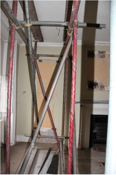
Metal work and damaged modern plaster finishes following removal of museum shelving, to be carefully removed and replaced with lath and plaster/original plaster to match existing adjacent.
