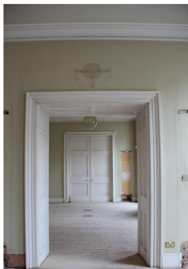
ELEVATION 1 - Metal work and damaged modern plaster finishes to be carefully removed and replaced with original plaster to match existing adjacent. Redecoration throughout. New FD30 double doors to be fitted in existing opening to match design of door 1-1-D01. Refer to detail drawing (32)AD002
