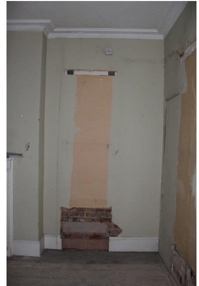
Metal work and damaged modern plaster finishes following removal of museum shelving, to be carefully removed and replaced with lath and plaster/original plaster to match existing adjacent.
