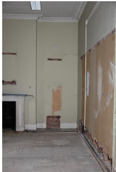
ELEVATION 5 - Metal work and damaged modern plaster finishes to be carefully removed and replaced with lath and plaster to match existing adjacent. Redecoration throughout.
