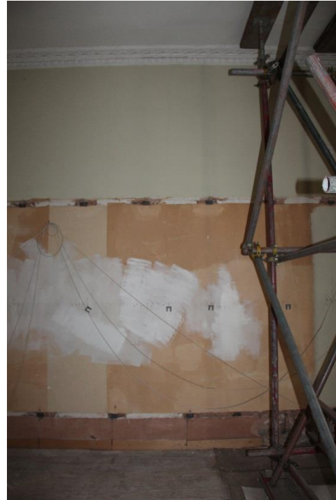
ELEVATION 7 - Metal work and damaged modern plaster finishes to be carefully removed and replaced with lath and plaster to match existing adjacent. Redecoration throughout. New enclosure design for main service run. Refer to BDP detail drawing (50)AD009
