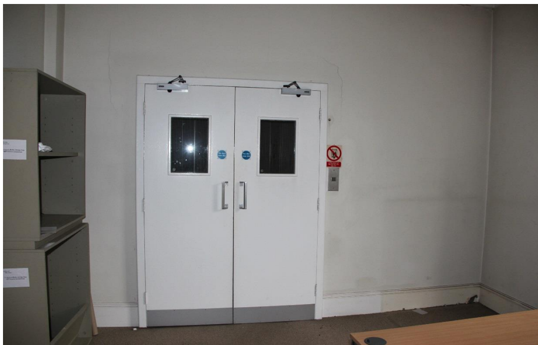
New internal door 1A-2-D02 to be fitted to match existing door 1A-2-D01, to replace existing lift shaft doors
