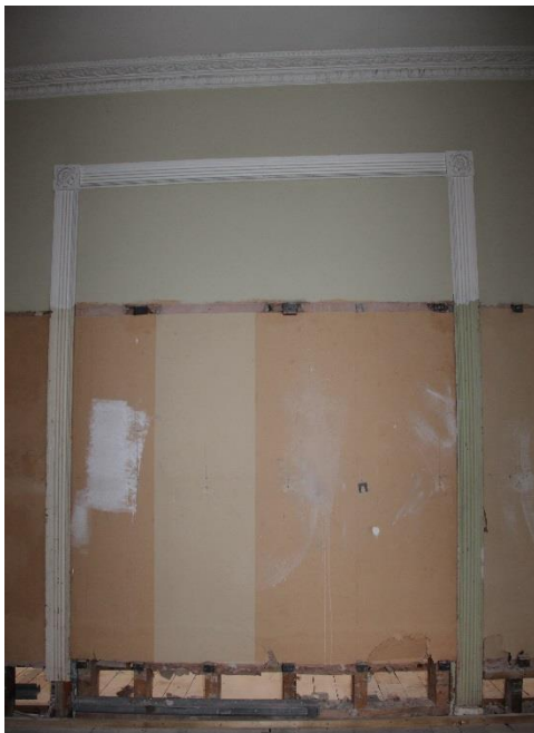
ELEVATION 6 - Original opening to be reinstated; Modern timber stud and plasterboard infill to be carefully removed; Fire upgrade requirements. Fire upgrade requirements. Damaged modern wall finishes to be made good to provide a suitable surface for new fire resistant board. Lath and plaster to be overboarded to achieve 30 minute fire protection. Existing cornice and skirting carefully removed, set aside with care and reinstated when the overboarding is completed. Ironmongery to be retained and refurbished.
