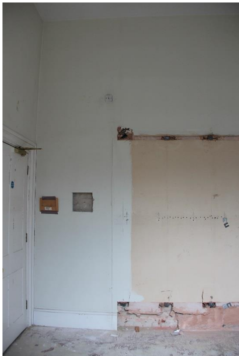
ELEVATION 6 - Metal work and damaged modern plaster finishes to be carefully removed and replaced with original plaster to match existing adjacent. Redecoration throughout.
