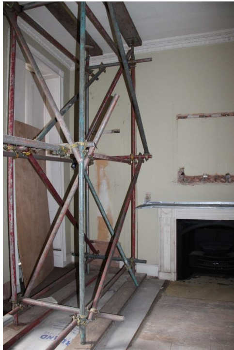
ELEVATION 5 - Metal work and damaged modern plaster finishes to be carefully removed and replaced with lath and plaster to match existing adjacent. Redecoration throughout.
