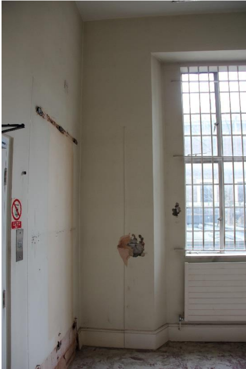
ELEVATION 5 - Damaged modern plaster finishes to be carefully removed and replaced with original plaster to match existing adjacent. Redecoration throughout. New sash window 1A-1-W04 to replace existing rear window. Refer to BDP drawing (31)AD002;
