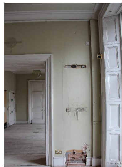
ELEVATION 1 - Metal work and damaged modern plaster finishes to be carefully removed and replaced with original plaster to match existing adjacent. Redecoration throughout. New FD30 double doors to be fitted in existing opening to match design of door 1-1-D01. Refer to detail drawing (32)AD002
