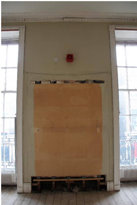
ELEVATION 2 - Windows and shutters to undergo full overhaul to ensure good working condition and receive full redecoration. Metal work and damaged modern plaster finishes to be carefully removed and replaced with lath and plaster to match existing adjacent. Redecoration throughout.
