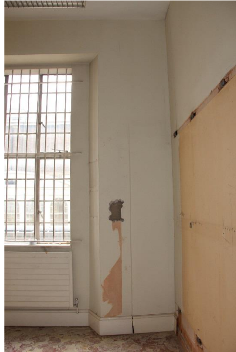
ELEVATION 5 - Damaged modern plaster finishes to be carefully removed and replaced with original plaster to match existing adjacent. Redecoration throughout. New sash window 1A-1-W04 to replace existing rear window. Refer to BDP drawing (31)AD002;
