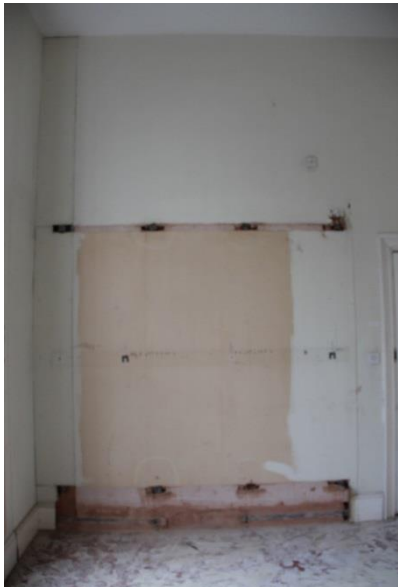
ELEVATION 1 - Metal work and damaged modern plaster finishes to be carefully removed. To be confirmed on site if wall provides 30 min fire resistance. If it doesn't, wall to be overboarded with new fire resistant board to provide the required 30 minute fire protection. If it does, damaged plasterboard replaced with plasterboard to match existing adjacent. Redecoration throughout. Existing door containing asbestos to be replaced with new FD30 door.
