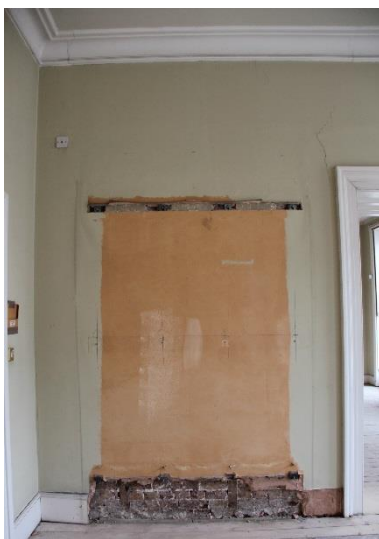
ELEVATION 1 - Metal work and damaged modern plaster finishes to be carefully removed and replaced with original plaster to match existing adjacent. Redecoration throughout. New FD30 double doors to be fitted in existing opening to match design of door 1-1-D01. Refer to detail drawing (32)AD002
