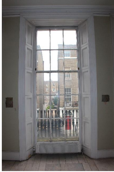
ELEVATION 2 - Windows and shutters to undergo full overhaul to ensure good working condition and receive full redecoration. Metal work and damaged modern plaster finishes to be carefully removed and replaced with original plaster to match existing adjacent. Redecoration throughout.
