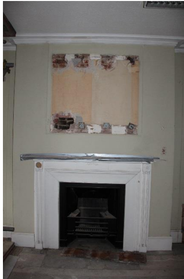
Metal work and damaged modern plaster finishes following removal of museum shelving, to be carefully removed and replaced with lath and plaster/original plaster to match existing adjacent.
