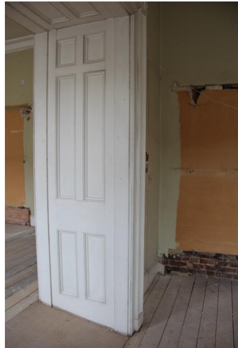
ELEVATION 2 – New FD30 double doors to be fitted in existing opening to match design of door 1-1-D01. Refer to detail drawing (32)AD002
