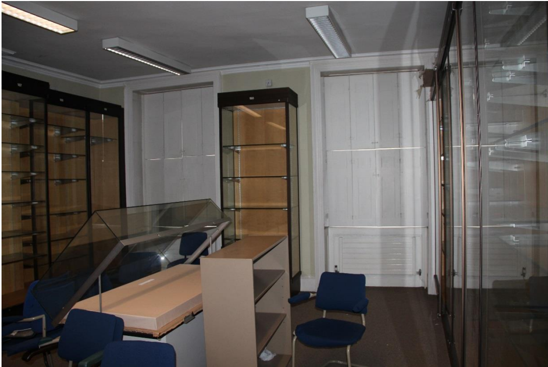
Windows and shutters to undergo full overhaul to ensure good working condition and receive full redecoration.
