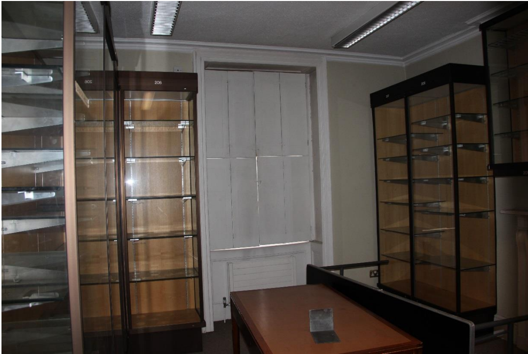
Windows and shutters to undergo full overhaul to ensure good working condition and receive full redecoration.
