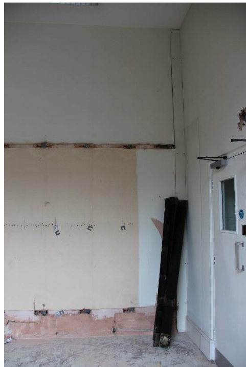
ELEVATION 6 - Metal work and damaged modern plaster finishes to be carefully removed and replaced with original plaster to match existing adjacent. Redecoration throughout.
