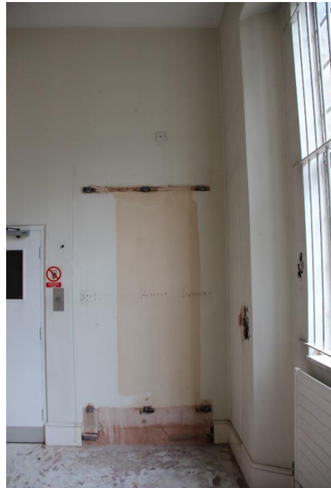
ELEVATION 3 - Metal work and damaged modern plaster finishes to be carefully removed and replaced with original plaster to match existing adjacent. Redecoration throughout. New FD30 double doors to replace existing lift shaft doors to match design of adjacent doors. Refer to detail drawing (32)AD002
