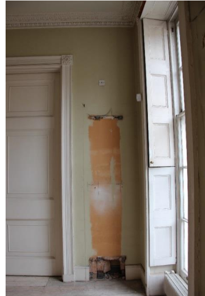
ELEVATION 3 - Damaged modern wall finishes to be carefully removed with existing adjacent construction to be made good. New lath and plaster finishes required and full redecoration throughout. Existing door to be refurbished and redecorated. Ironmongery to be retained and refurbished.
