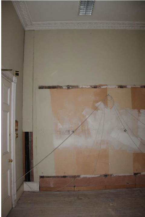
ELEVATION 7 - Metal work and damaged modern plaster finishes to be carefully removed and replaced with lath and plaster to match existing adjacent. Redecoration throughout. New enclosure design for main service run. Refer to BDP detail drawing (50)AD009
