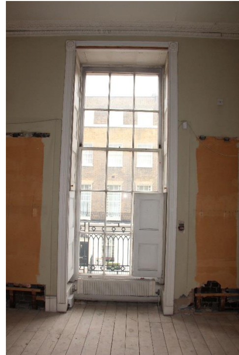
ELEVATION 2 - Windows and shutters to undergo full overhaul to ensure good working condition and receive full redecoration. Metal work and damaged modern plaster finishes to be carefully removed and replaced with lath and plaster to match existing adjacent. Redecoration throughout.
