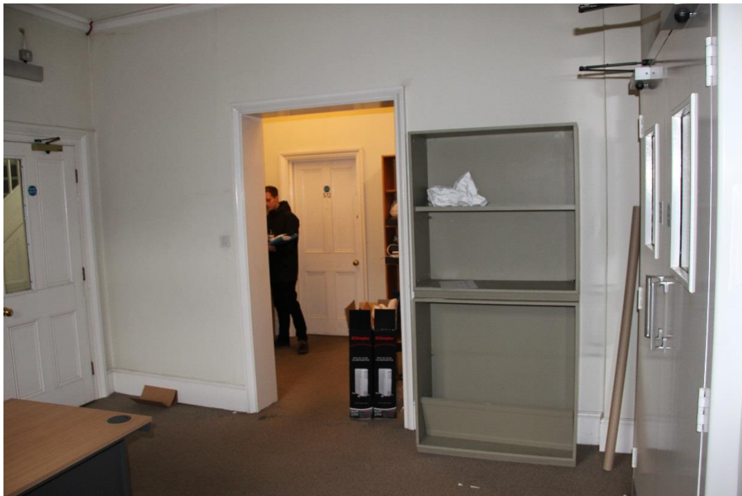
Existing opening to be retained. Redecoration throughout;
