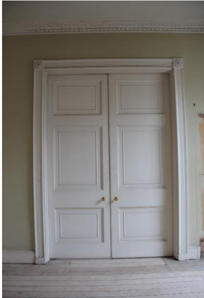
ELEVATION 3 - Damaged modern wall finishes to be carefully removed with existing adjacent construction to be made good. New lath and plaster finishes required and full redecoration throughout. Existing door to be refurbished and redecorated. Ironmongery to be retained and refurbished.
