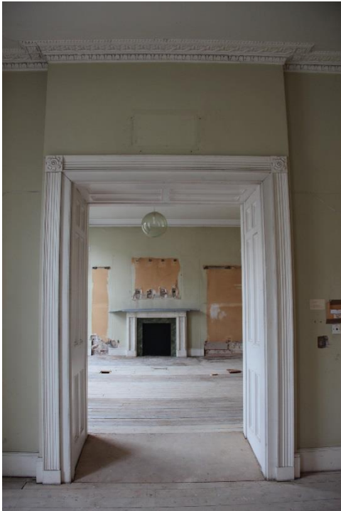
ELEVATION 2 – New FD30 double doors to be fitted in existing opening to match design of door 1-1-D01. Refer to detail drawing (32)AD002
