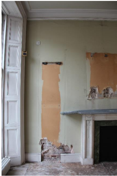
ELEVATION 3 - Metal work and damaged modern plaster finishes to be carefully removed and replaced with original plaster to match existing adjacent. Redecoration throughout. Existing door containing asbestos to be replaced with new FD30 door.
