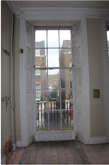
ELEVATION 2 - Windows and shutters to undergo full overhaul to ensure good working condition and receive full redecoration. Metal work and damaged modern plaster finishes to be carefully removed and replaced with original plaster to match existing adjacent. Redecoration throughout.
