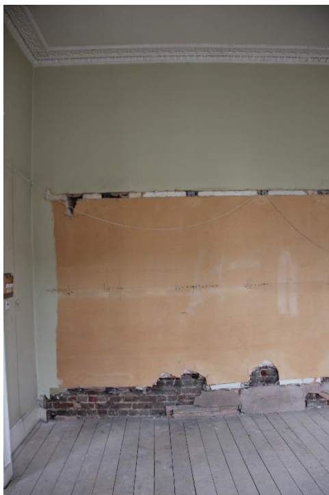
ELEVATION 2 – New FD30 double doors to be fitted in existing opening to match design of door 1-1-D01. Refer to detail drawing (32)AD002
