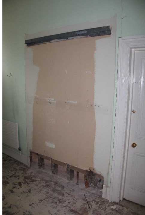
Damaged modern plaster finishes to be carefully removed and replaced with plasterboard to match existing adjacent. Redecoration throughout.
