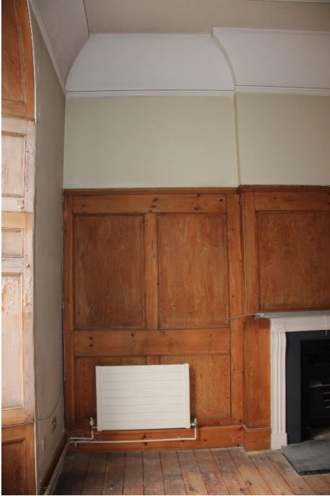
ELEVATION 3 - Existing radiators to be carefully removed with all other existing services. Original timber panelling to front elevation to be retained, refurbished and redecorated.
