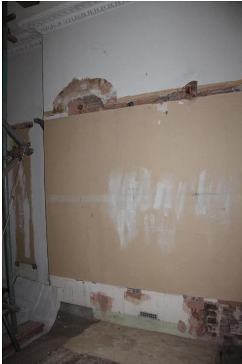
ELEVATION 1 - Metal work and damaged modern plaster finishes to be carefully removed and replaced with lath and plaster to match existing adjacent. Redecoration throughout.
