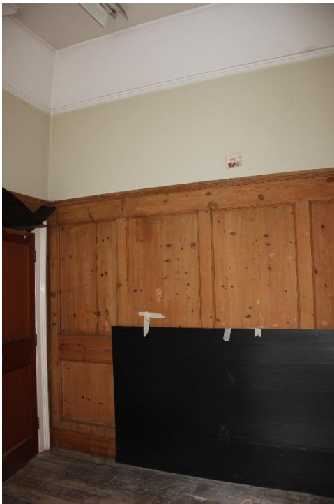
ELEVATION 4 - Original timber panelling to front elevation to be retained, refurbished and redecorated
