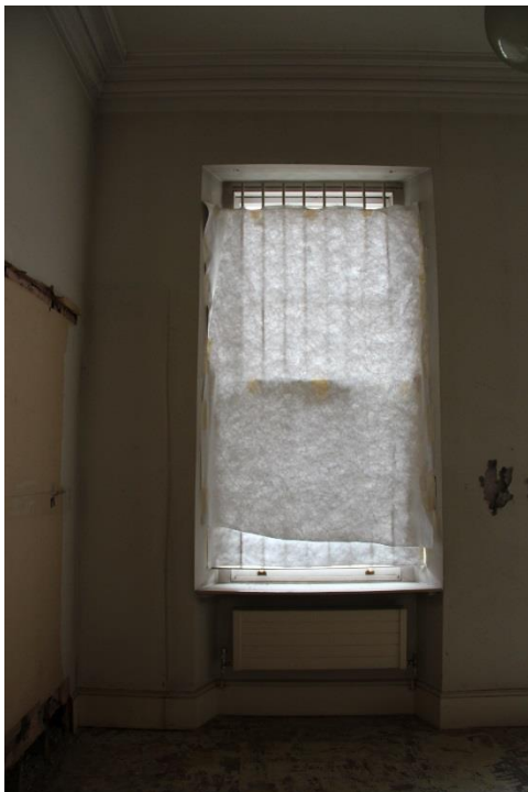
ELEVATION 2 - Existing radiators to be carefully removed with all other existing services. Windows to undergo full overhaul to ensure good working condition and receive full redecoration
