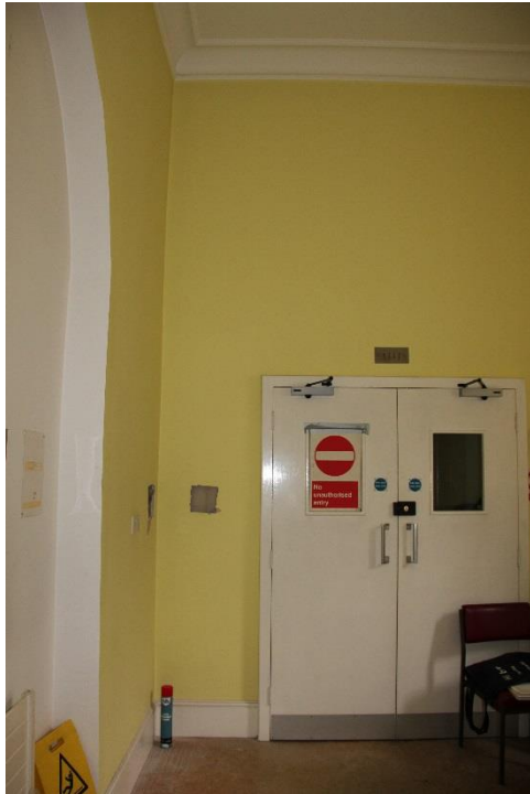
ELEVATION 3 - Existing lift shaft doors to be carefully removed and replaced with new doors to match design of adjacent doors. See BDP drawing (32)AD002. Existing external door containing asbestos to be replaced with new door to match design of existing. Refer to BDP drawing (32)AD001
