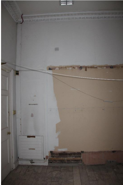
ELEVATION 3 - Metal work and damaged modern plaster finishes to be carefully removed and replaced with lath and plaster to match existing adjacent. Redecoration throughout.
