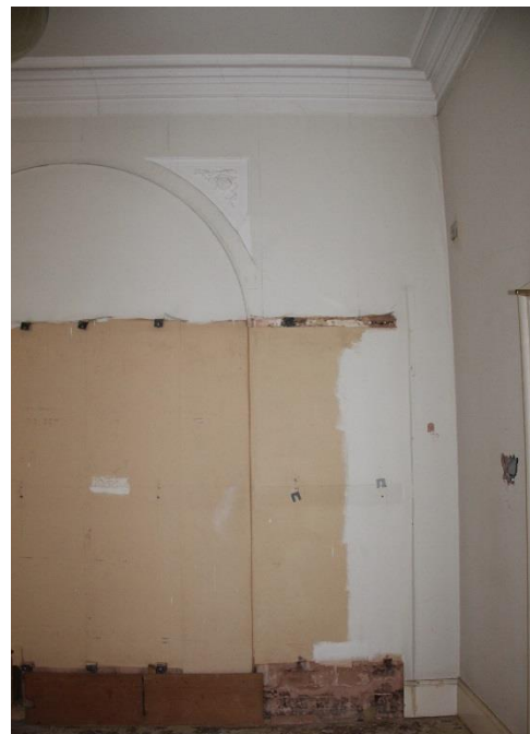
ELEVATION 4 - Modern timber stud and plasterboard infill to be carefully removed to reinstate original opening. New replacement plasterboard finish to damaged areas of walls and redecoration throughout.
