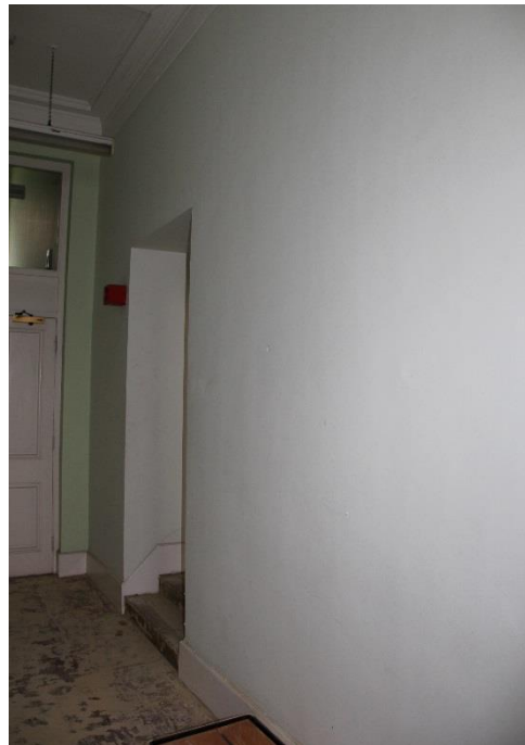
Damaged modern plaster finishes to be carefully removed and replaced with plasterboard to match existing adjacent. Redecoration throughout.
