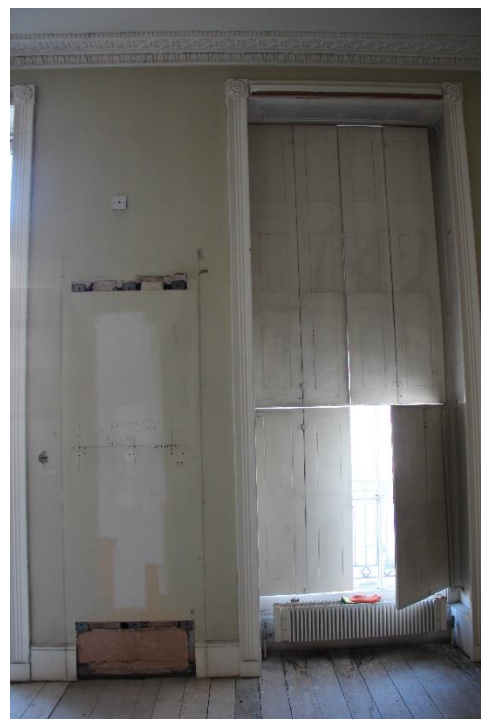
ELEVATION 2 - Metal work and damaged modern plaster finishes to be carefully removed and replaced with lath and plaster to match existing adjacent. Windows and shutters to undergo full overhaul to ensure good working condition and receive full redecoration. Redecoration throughout.
