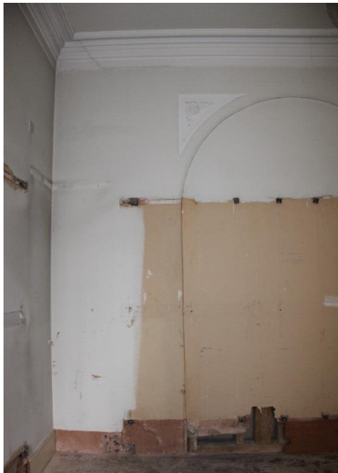
ELEVATION 4 - Modern timber stud and plasterboard infill to be carefully removed to reinstate original opening. New replacement plasterboard finish to damaged areas of walls and redecoration throughout.
