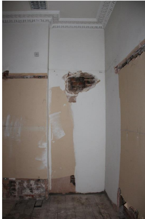
ELEVATION 1 - Metal work and damaged modern plaster finishes to be carefully removed and replaced with lath and plaster to match existing adjacent. Redecoration throughout.
