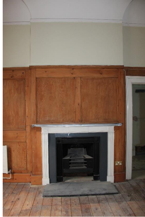
ELEVATION 3 - Existing radiators to be carefully removed with all other existing services. Original timber panelling to front elevation to be retained, refurbished and redecorated.
