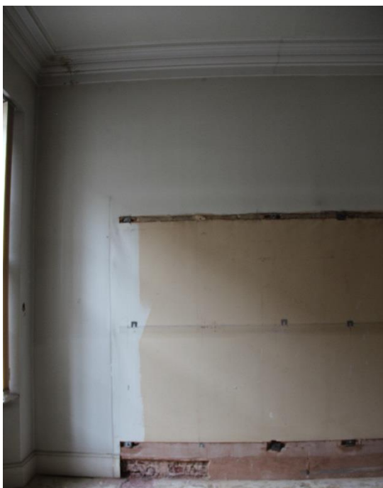
ELEVATION 3 - Metal work and damaged modern plaster finishes to be carefully removed and replaced with plasterboard to match existing adjacent. Redecoration throughout.
