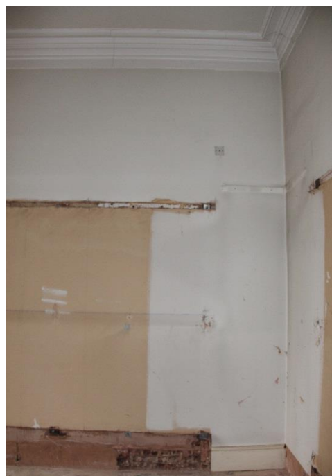
ELEVATION 3 - Metal work and damaged modern plaster finishes to be carefully removed and replaced with plasterboard to match existing adjacent. Redecoration throughout.
