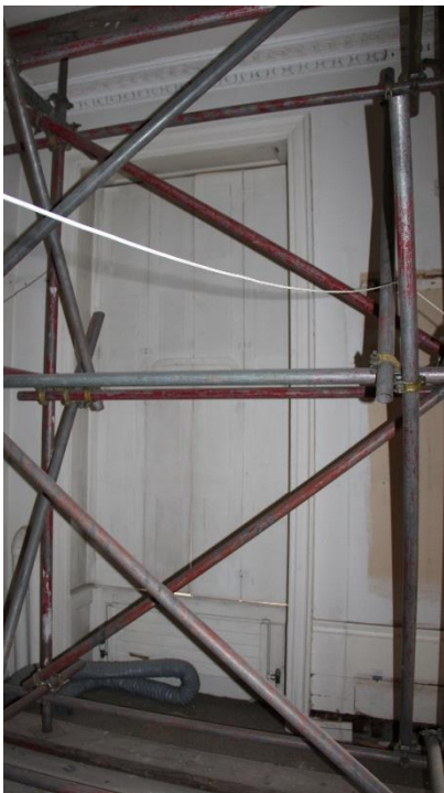
ELEVATION 4 - Existing radiators to be carefully removed with all other existing services. Original timber panelling to front elevation to be retained, refurbished and redecorated. Windows to undergo full overhaul to ensure good working condition and receive full redecoration
