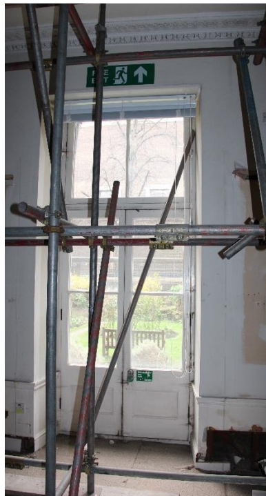
ELEVATION 4 - Existing radiators to be carefully removed with all other existing services. Original timber panelling to front elevation to be retained, refurbished and redecorated. Windows to undergo full overhaul to ensure good working condition and receive full redecoration
