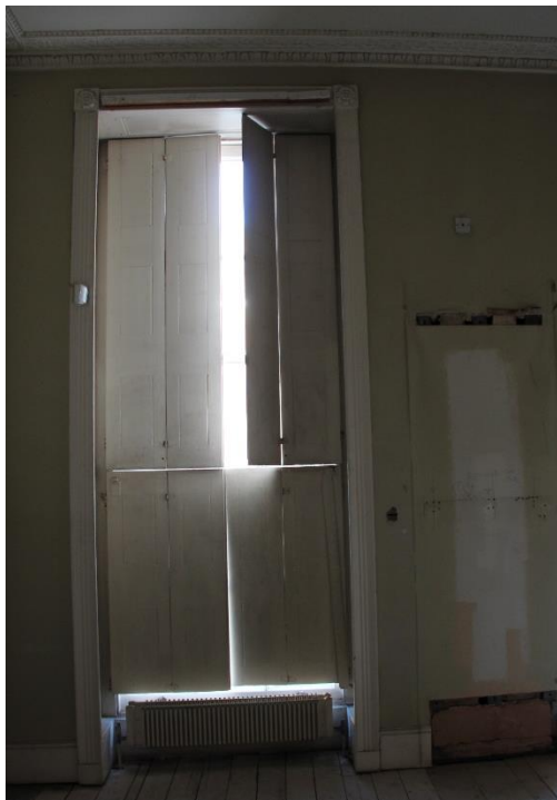
ELEVATION 2 - Metal work and damaged modern plaster finishes to be carefully removed and replaced with lath and plaster to match existing adjacent. Windows and shutters to undergo full overhaul to ensure good working condition and receive full redecoration. Redecoration throughout.
