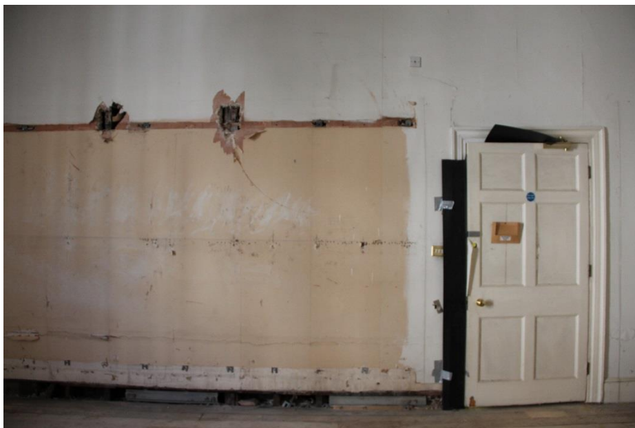
ELEVATION 4 - Existing door refurbished and redecorated. Fire upgrade requirements. Damaged modern wall finishes to be made good to provide a suitable surface for new fire resistant board. Lath and plaster to be overboarded to achieve 30 minute fire protection. Existing cornice and skirting carefully removed, set aside with care and reinstated when the overboarding is completed. Ironmongery to be retained and refurbished.
