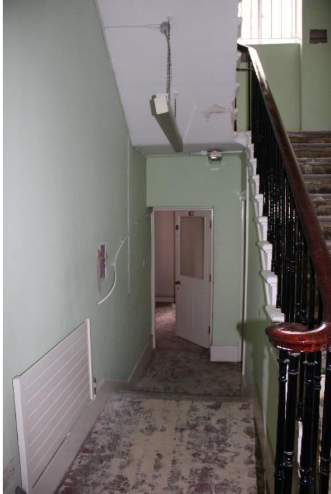
Existing door containing asbestos underneath stairs to basement, to be replaced with new door to match design of existing. Refer to BDP drawing (32)AD001
