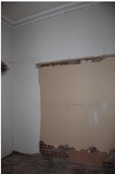
ELEVATION 2 - Damaged modern wall finishes to be carefully removed with existing adjacent construction to be made good. New lath and plaster finishes required and full redecoration throughout. Existing door refurbished and redecorated. Fire upgrade requirements TBD. Ironmongery to be retained and refurbished.
