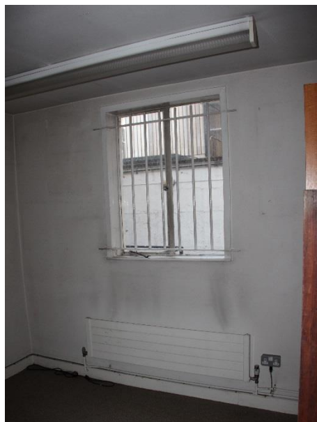
Door to be replaced to comply with fire escape strategy. Metal framed window refurbished in situ. Redecoration required throughout.
