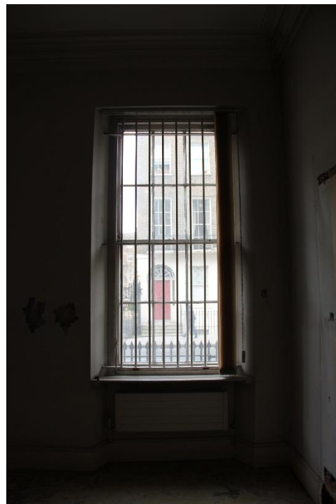
ELEVATION 2 - Existing radiators to be carefully removed with all other existing services. Windows to undergo full overhaul to ensure good working condition and receive full redecoration
