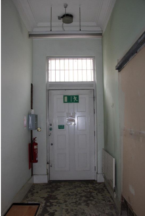
Damaged modern plaster finishes to be carefully removed and replaced with plasterboard to match existing adjacent. Redecoration throughout.
