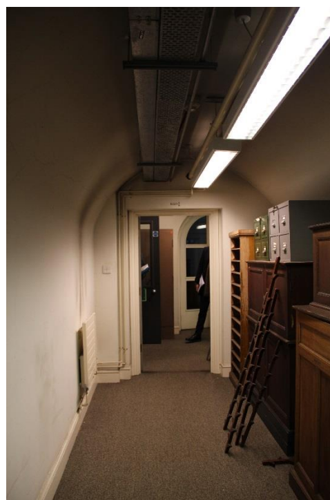
New plasterboard stud partition with plaster finish to be formed to create shower enclosure and lobby area within existing room
