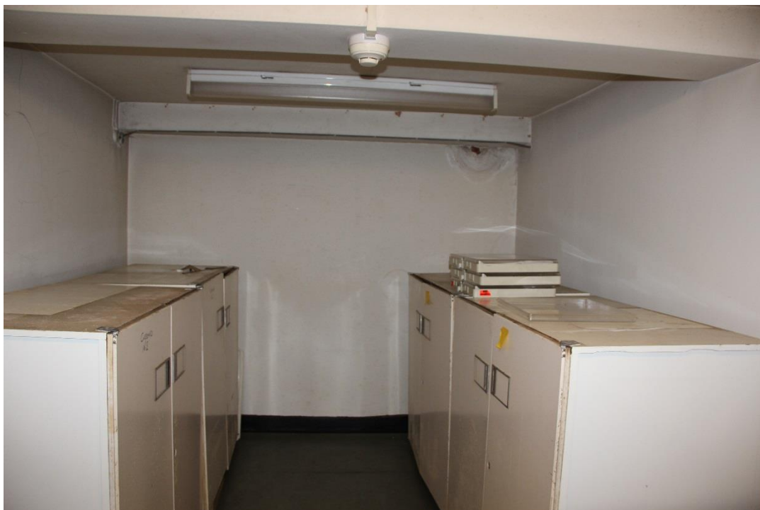
Two new openings to be made in existing wall to enlarge room to accommodate toilets and shower
