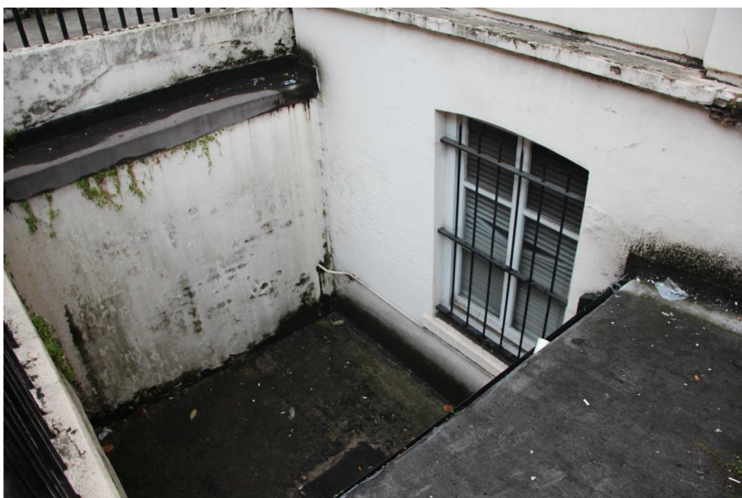
Vegetation to be removed from flat asphalt roof and repairs to be carried out where necessary
