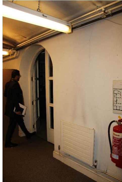
New ceiling bulkheads required to run each side of the ceiling to contain incoming services.
