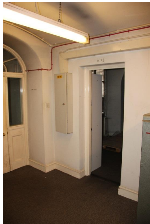
New ceiling bulkheads required to run each side of the ceiling to contain incoming services.
