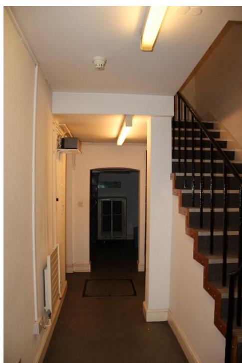
Stairs and lobby area to be redecorated; New door to be fitted in opening to space under stairs to create store room
