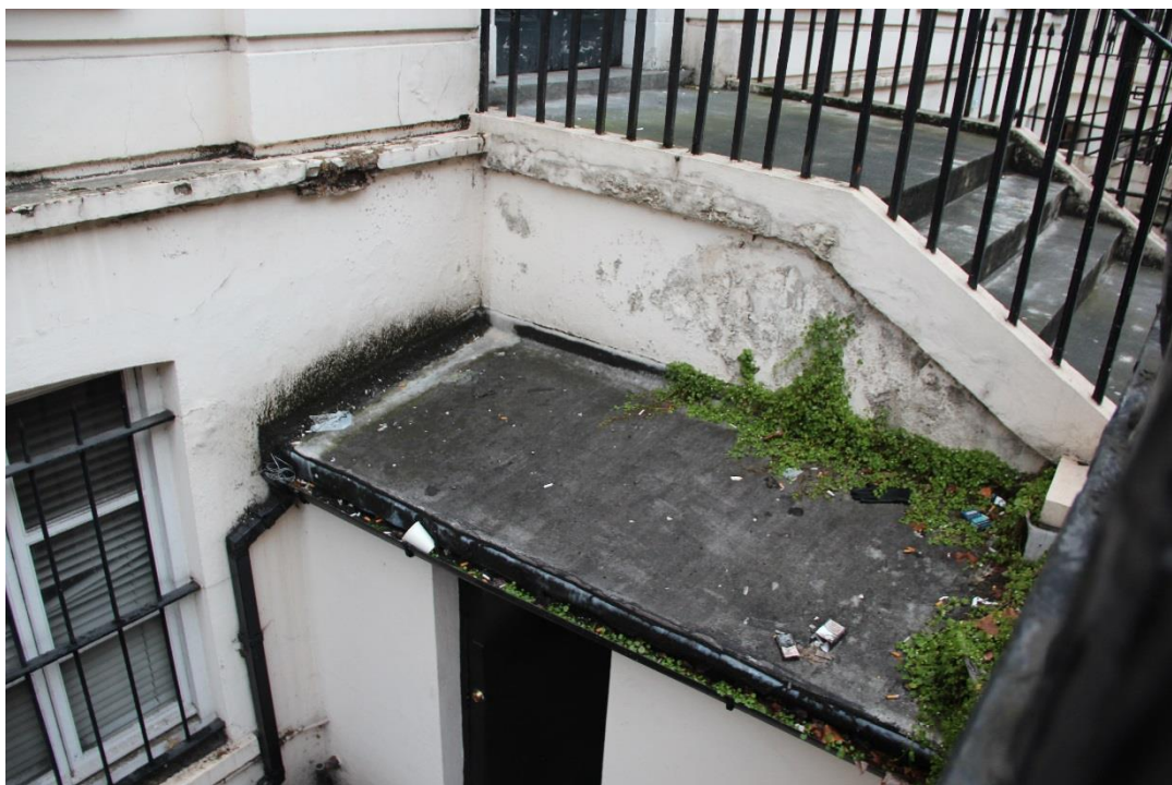
Vegetation to be removed from flat asphalt roof and repairs to be carried out where necessary
