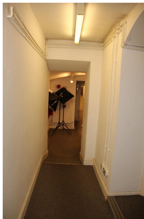
New door to be installed in existing opening linking 1MS to 1AMS
