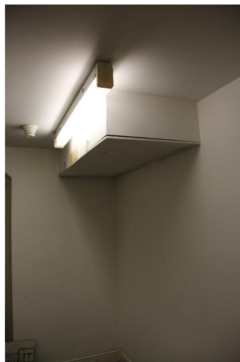
New suspended ceiling to be installed to conceal new services and decorated in matt emulsion paint;
