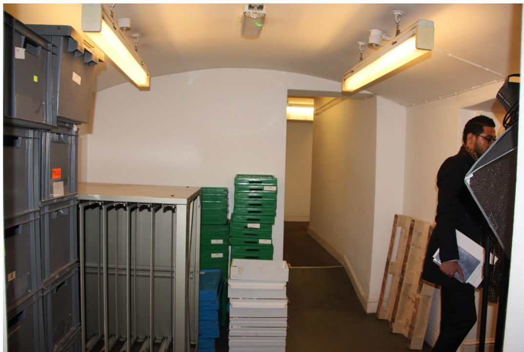
New door to be fitted in opening in party wall linking 1MS to 1AMS
