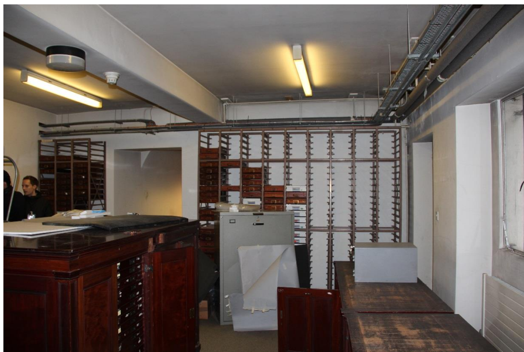
Existing windows, doors, floor, ceiling and walls to be redecorated
