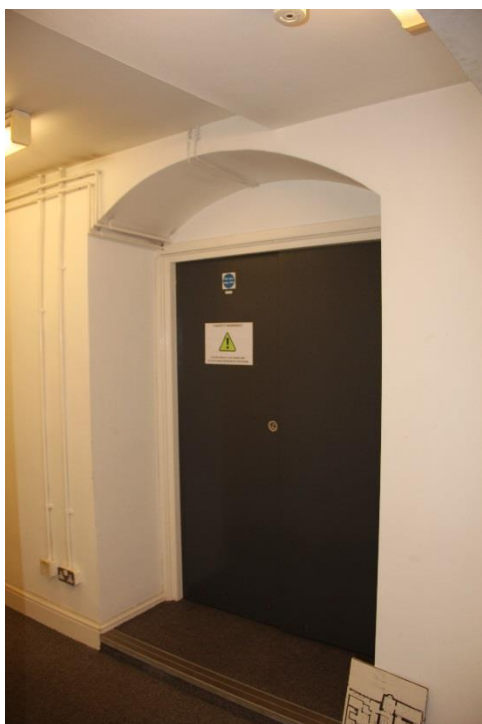
Existing doors retained to be refurbished and redecorated
