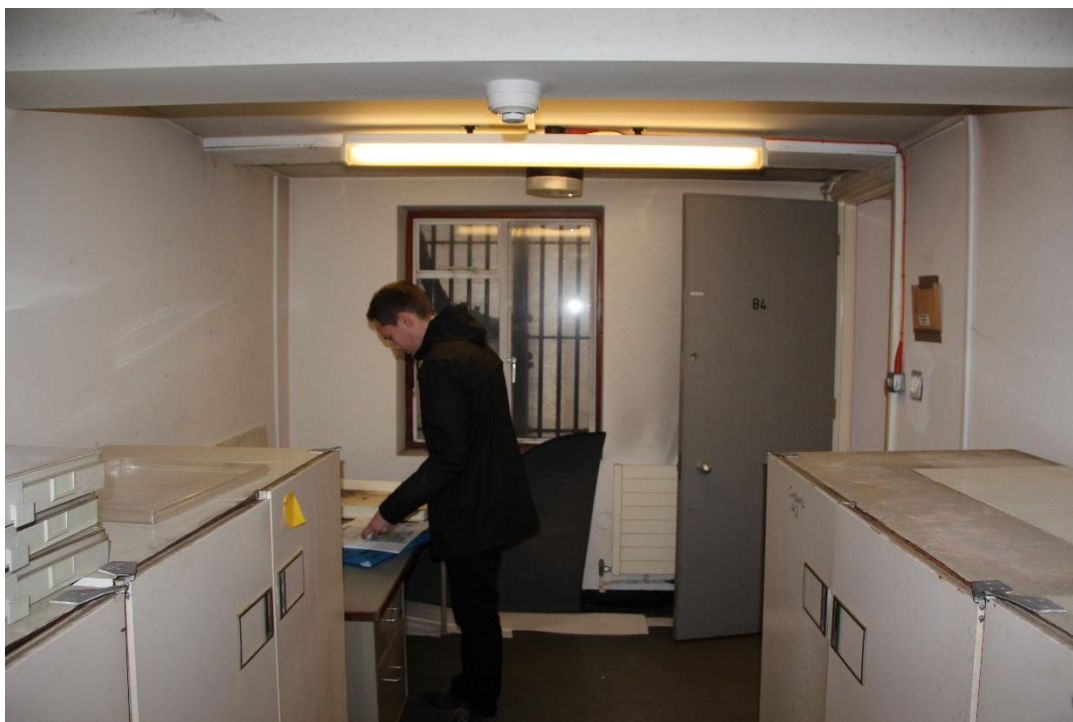
Existing door opening to be infilled to block existing link to adjoining room
