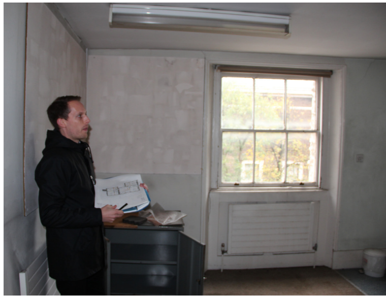
Existing room 1AMS/5/004
