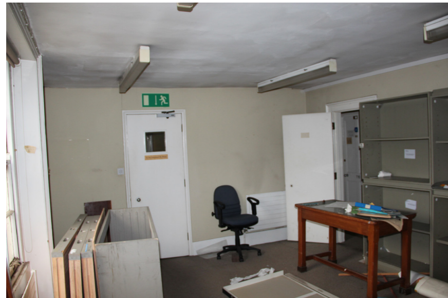
Existing room 1MS/5/012
