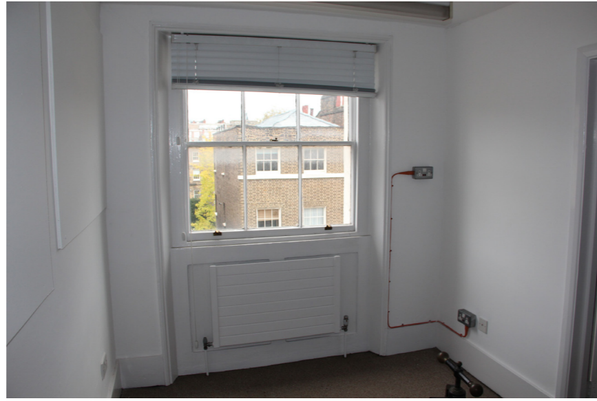
Existing room 1AMS/5/002
