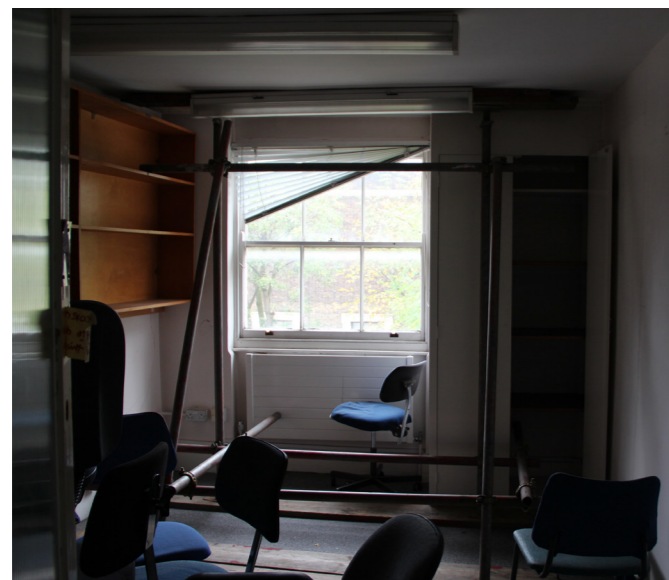
Existing room 1MS/5/013
