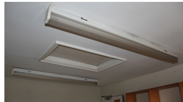
Existing room 1MS/5/011
