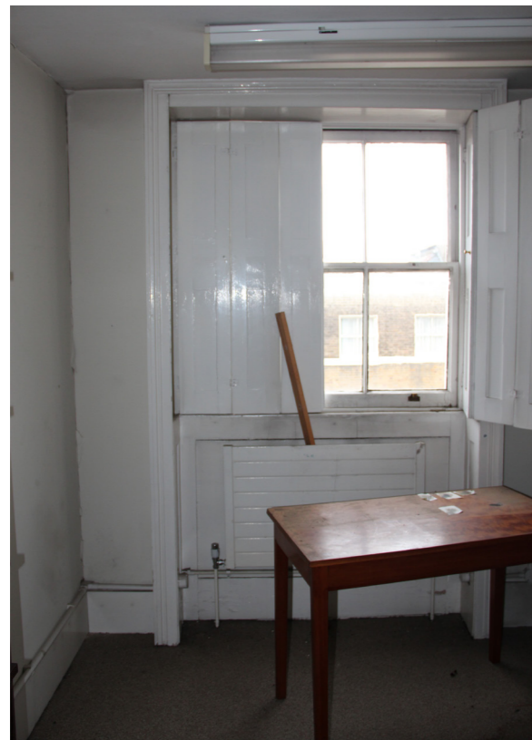
Existing room 1MS/5/010
