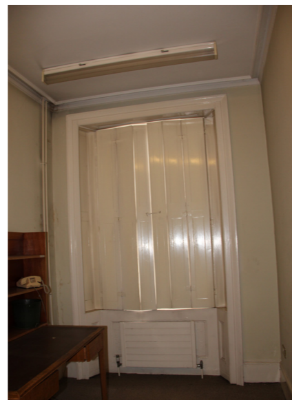
Existing room 1AMS/4/013
