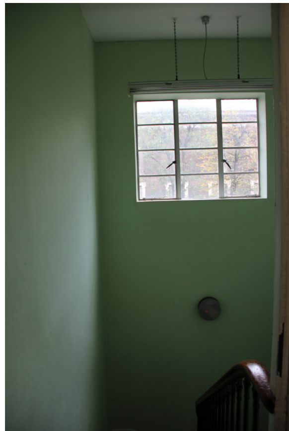
Existing room 1AMS/4/s02
