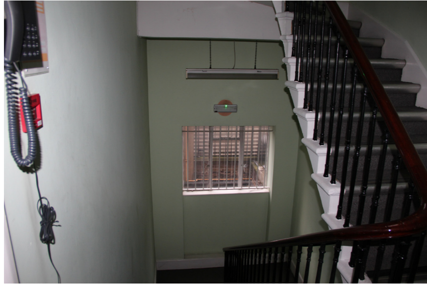
Existing room 1AMS/3/S01
