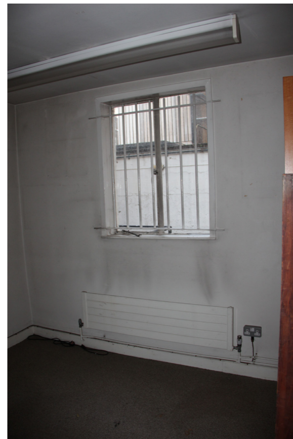
Existing room 1AMS/2/015
