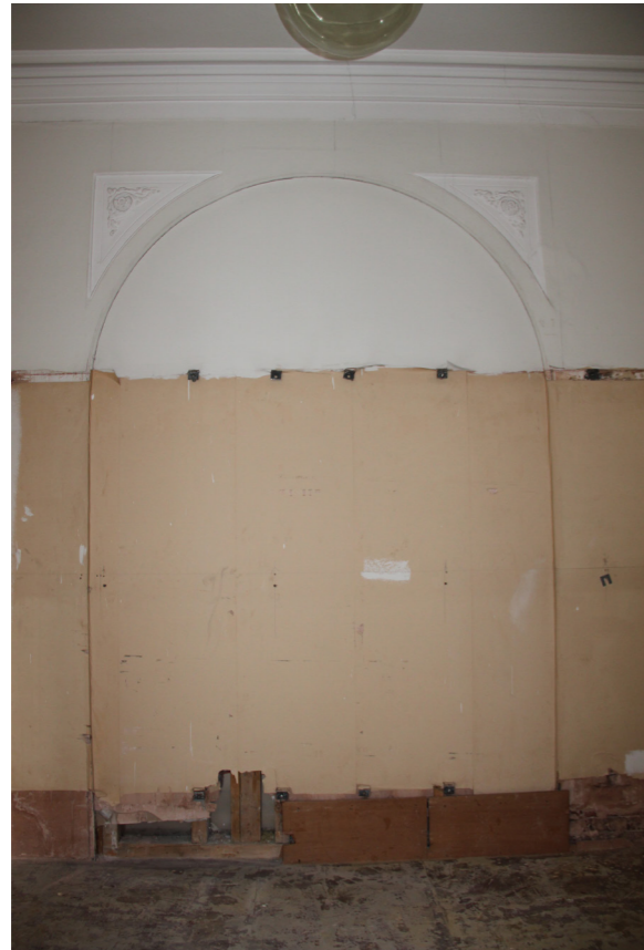
Existing room 1AMS/2/013
