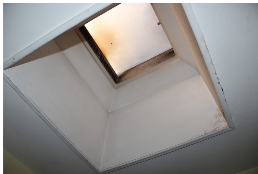
Existing room 1MS/2/007
