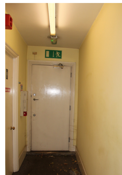
Existing room 1MS/2/009
