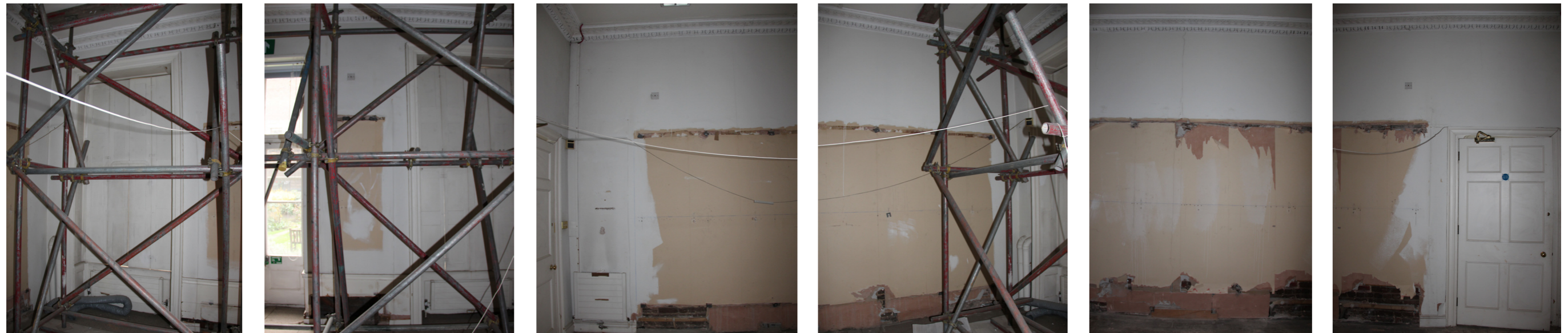
Existing room 1MS/2/006
