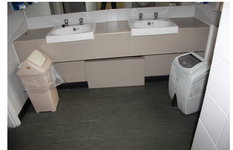
Existing room 1MS/2/010
