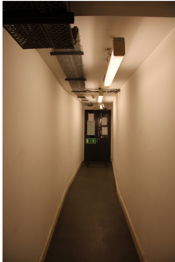
Existing room 1AMS Tunnel
