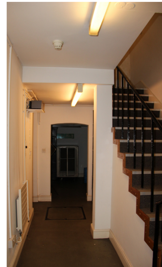
Existing room 1AMS/1/S01
