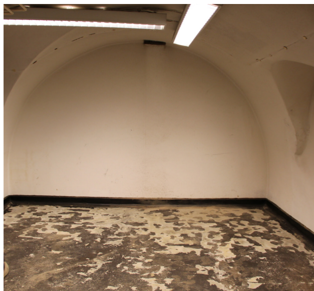
Existing room 1MS/1/019
