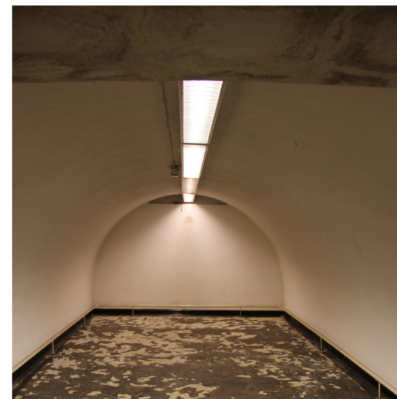
Existing room 1MS/1/020
