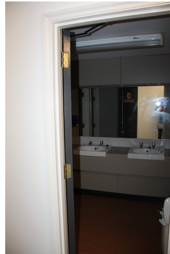
Existing room 1MS/1/018
