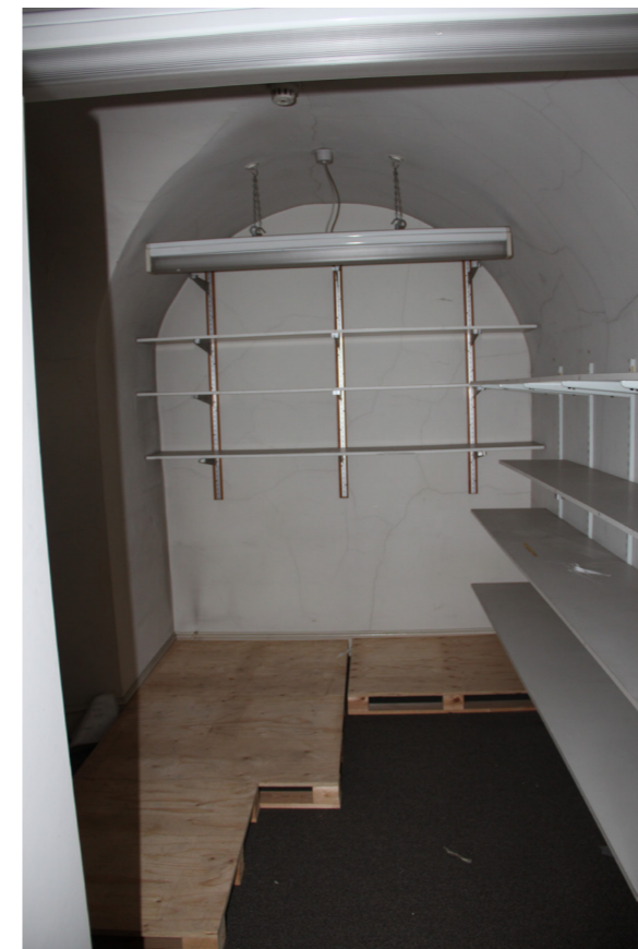
Existing room 1MS/1/012
