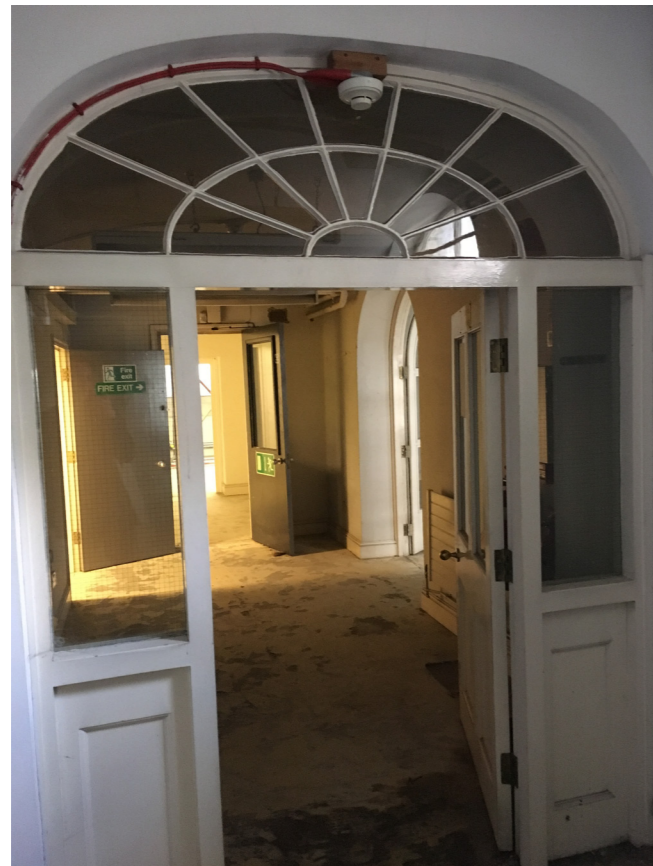
Existing room 1MS/1/011
