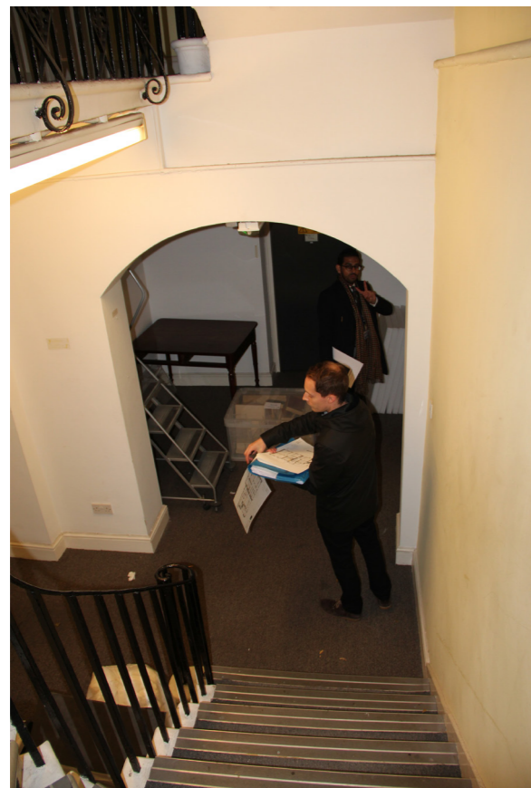
Existing room 1MS/1/021
