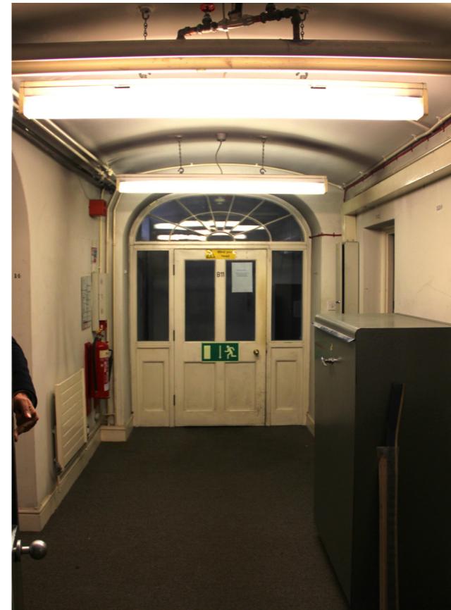
Existing room 1MS/1/010
