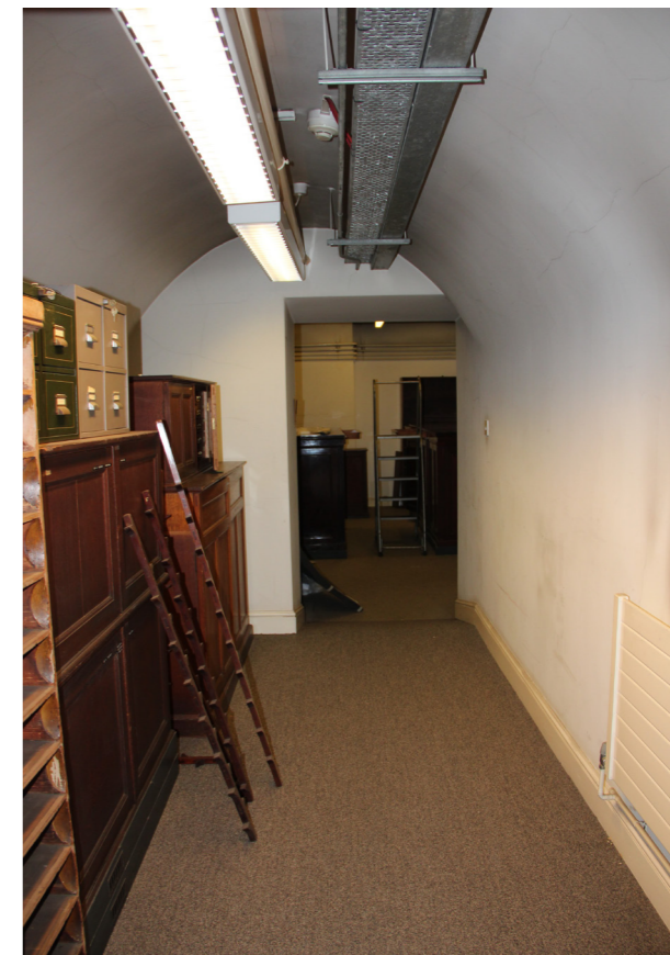
Existing room 1MS/1/013
