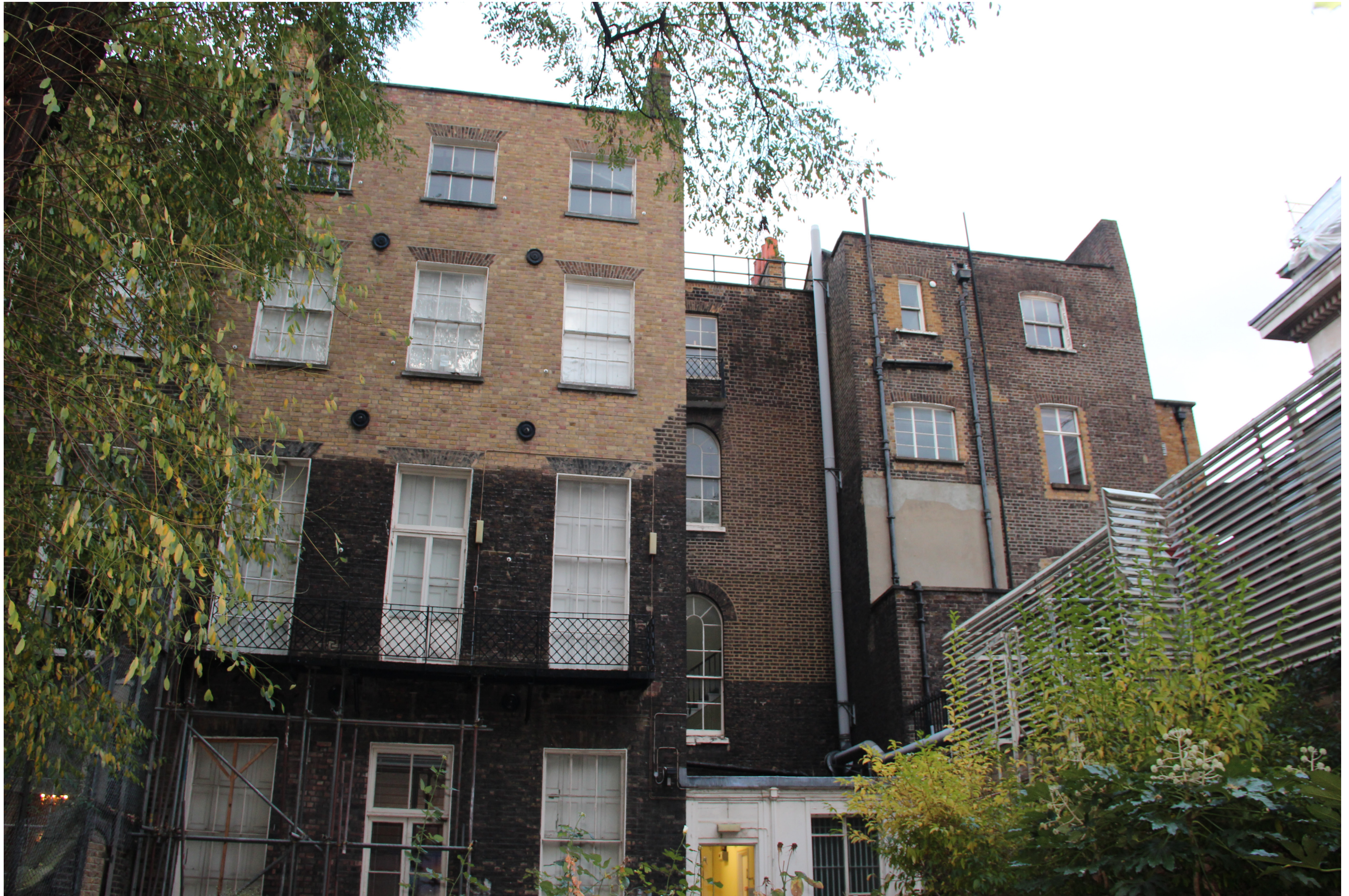
1 and 1A Montague Street Rear Elevation
