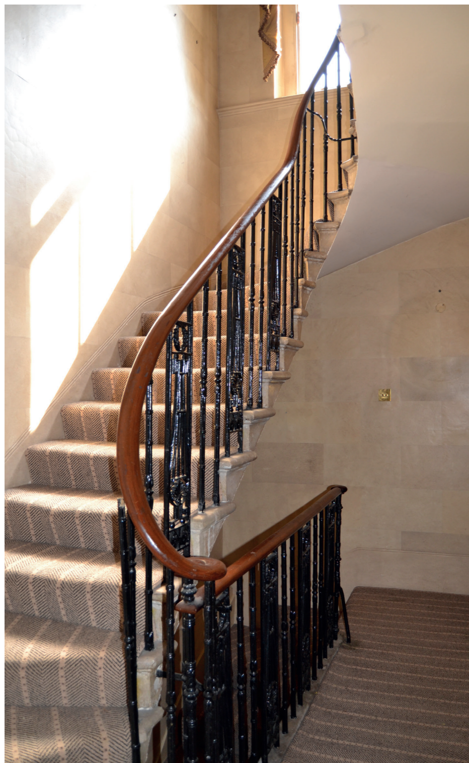
Figure 3.9 Cantilever stone staircase within Gloucester Lodge, thought to date from the Papworth subdivision of the villa.
