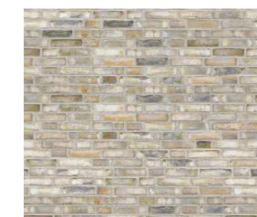
Brick to rear facade
