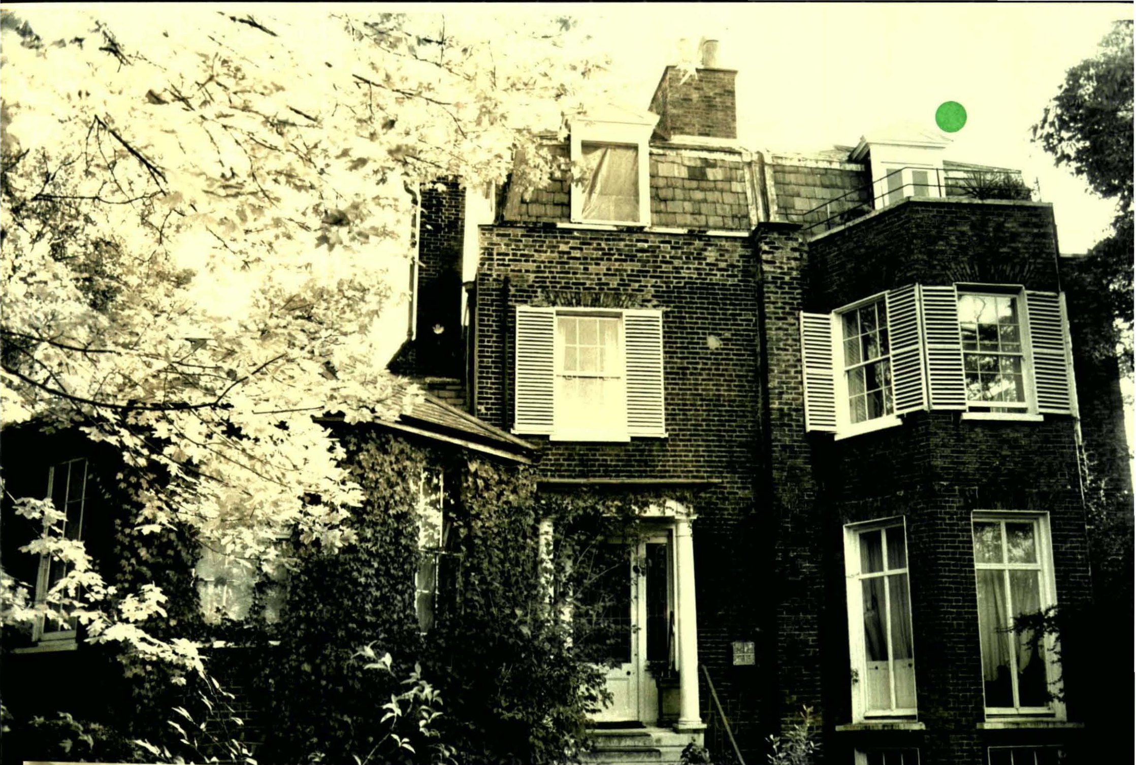
19, Frogmal Lane as seen from Chesterford Gardens Green dot marks window with proposed alterations
