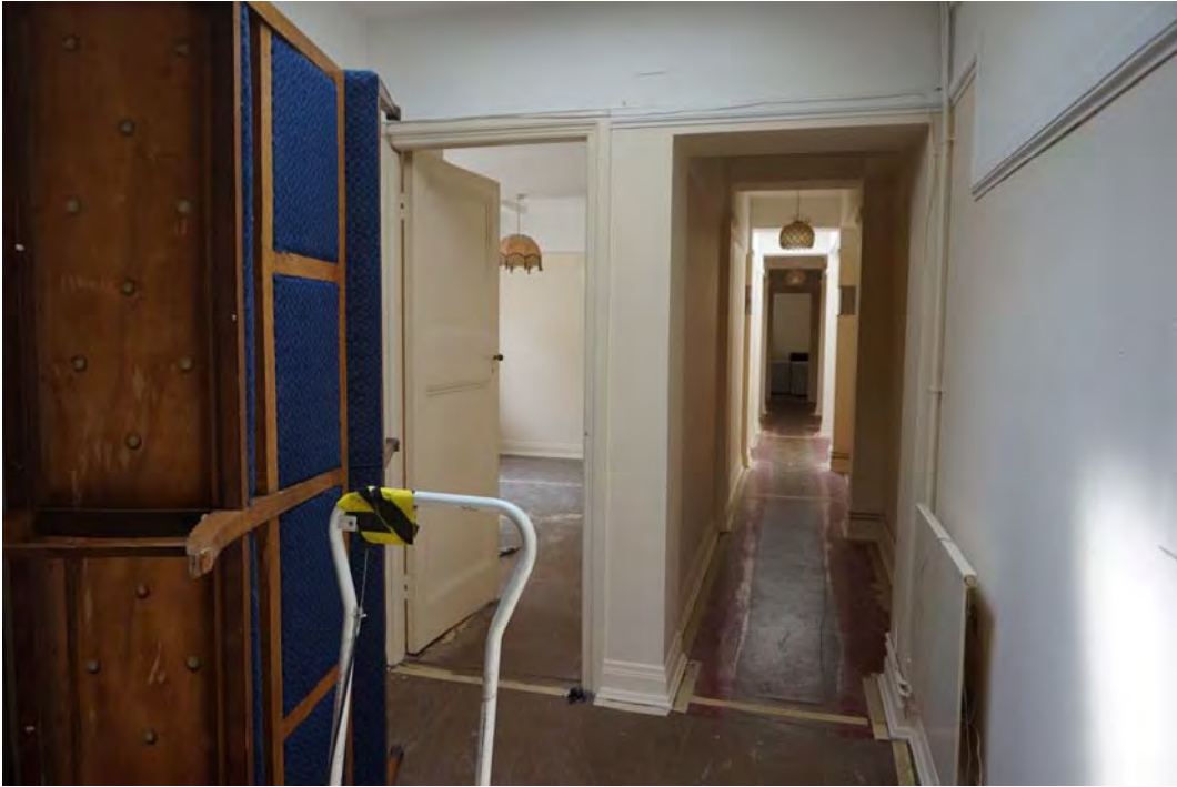
Figure 9: Internal corridor within apartment
