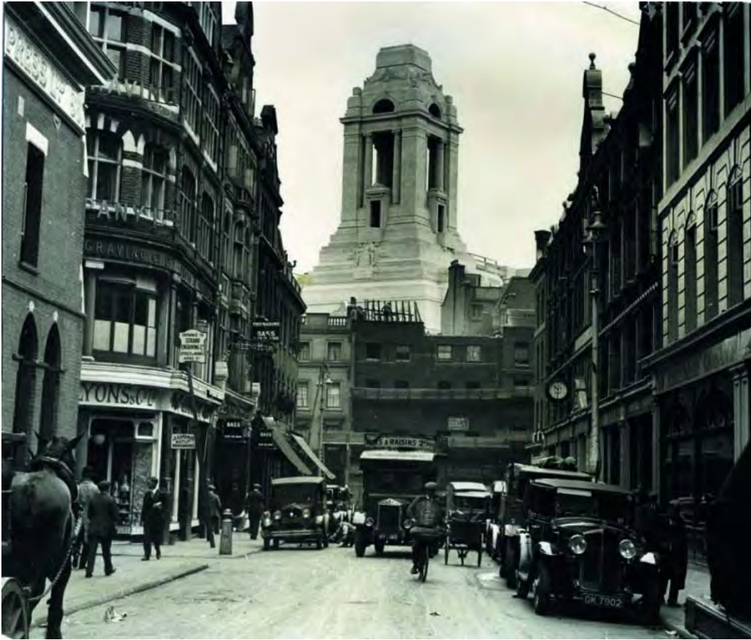
Figure 7: View over partially demolished buildings 1931 (©UGLE)
