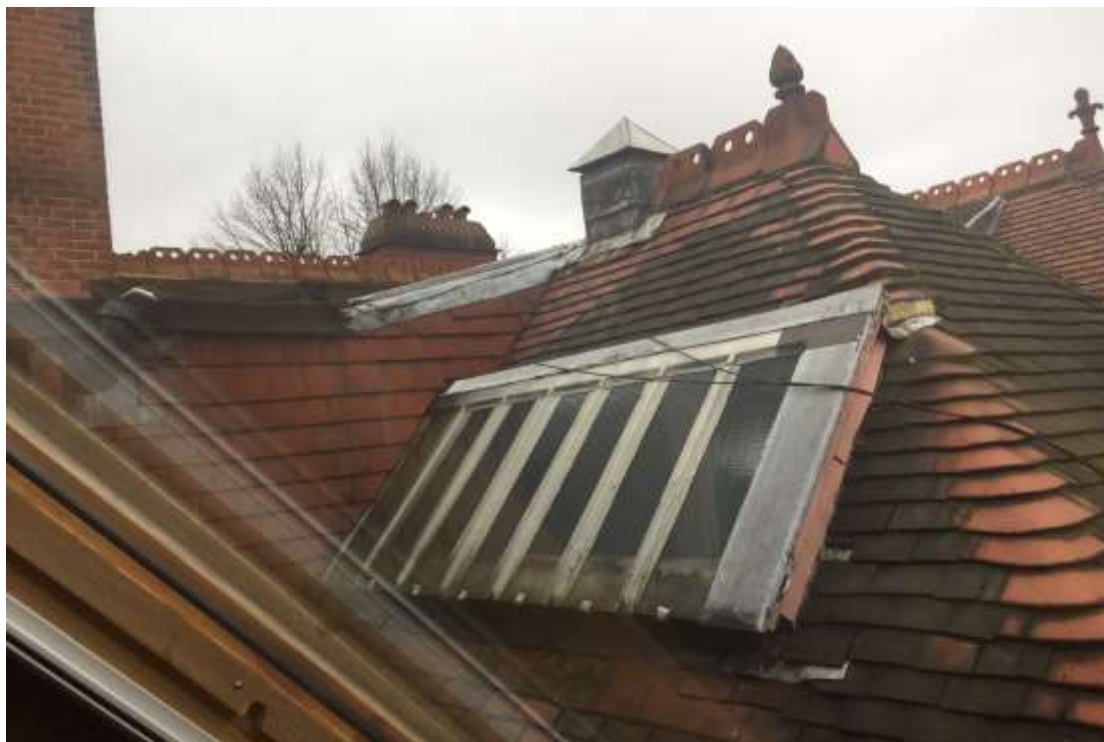
VIEW OF PART ROOF – ITEM a)
