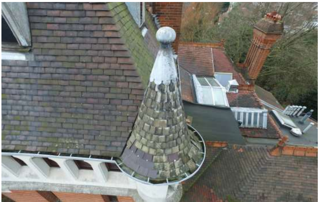
VIEW OF PART ROOF - ITEM h)
