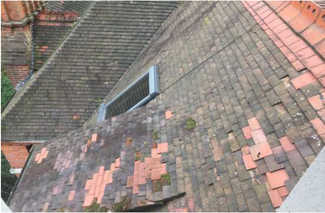
VIEW OF PART ROOF - ITEM c)
