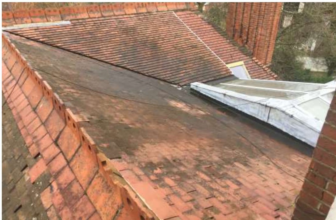
VIEW OF PART ROOF - ITEM e)
