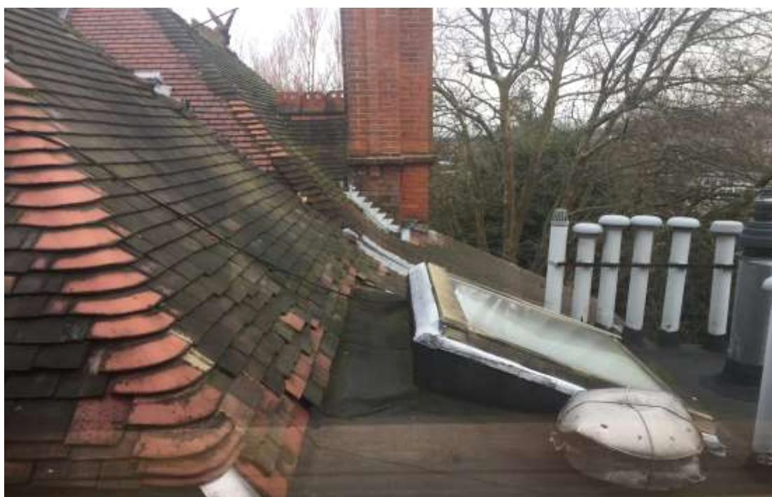
VIEW OF PART ROOF - ITEM b)
