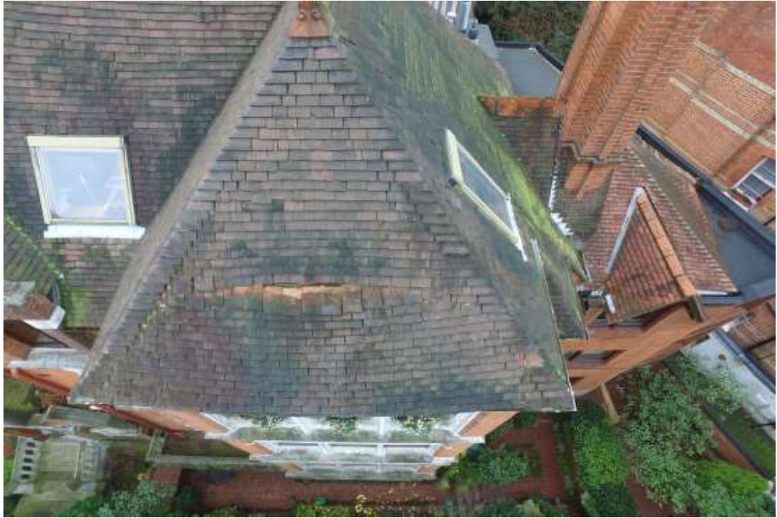
VIEW OF PART ROOF - ITEM i)
