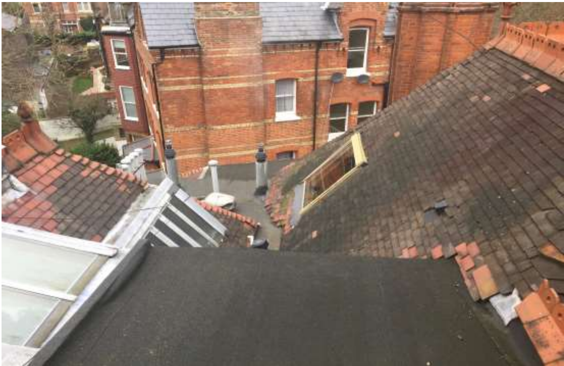
VIEW OF PART ROOF - ITEM d)
