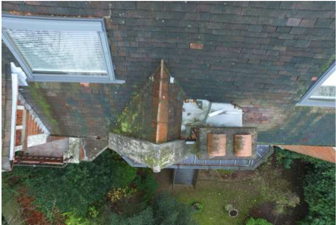
VIEW OF PART ROOF - ITEM g)
