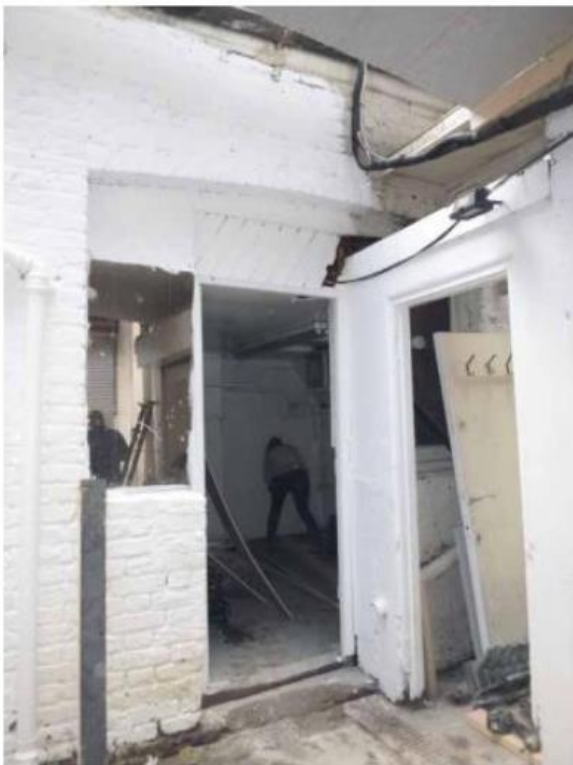
Above: Rear workshop building
