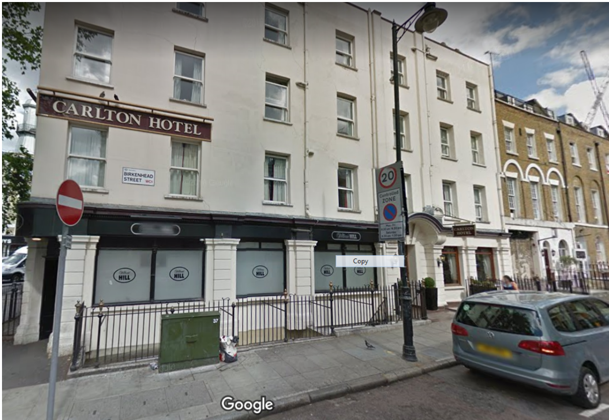
Photo 3 shows view of pre-existing site on Birkenhead Street elevation and adjacent listed terrace
