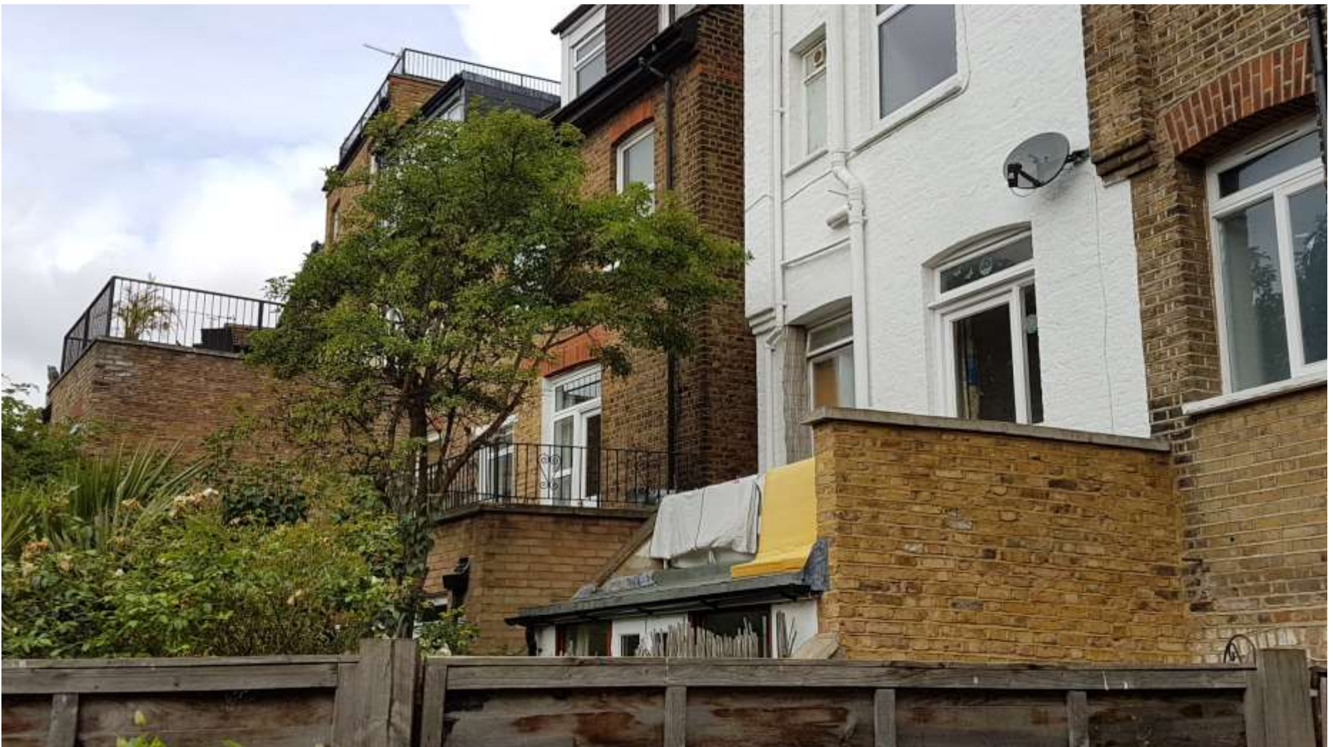
Existing Balconies to the rear of 120, 118 and 116 Mill Lane, NW6
