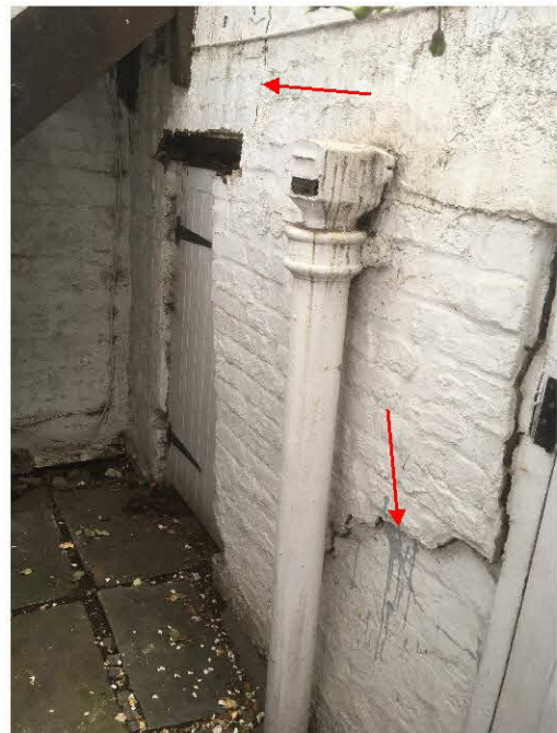
Figure 2: Note crack left of RH door
