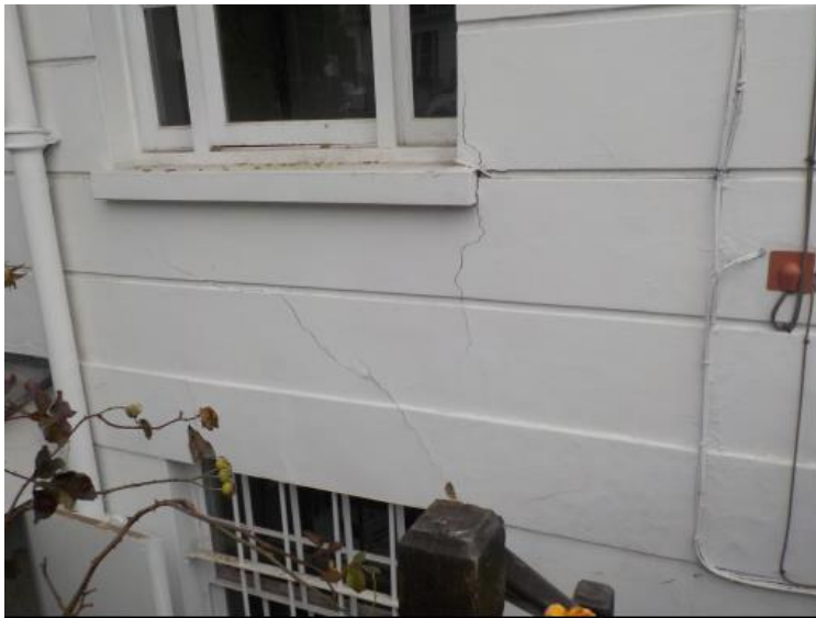
Between ground and lower ground floor window
