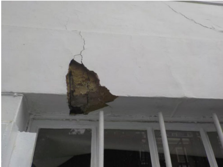
Lower ground floor window, partial rendering removed to expose that the concrete lintel is broken
