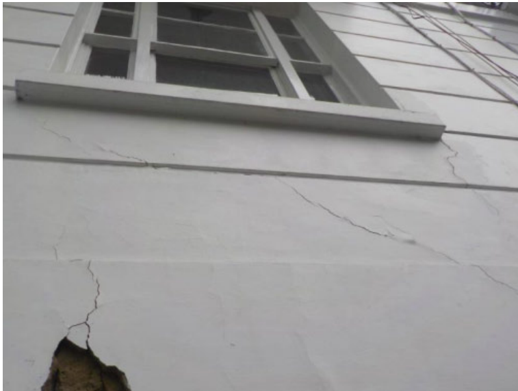
Between ground and lower ground floor window
