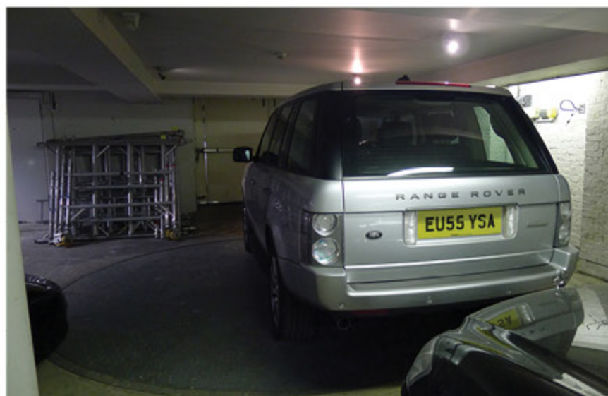
Car parked on the turntable providing increased manoeuvrability and removing the need for the car to reverse onto to the street.
