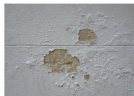
Photograph of the facade with faux-stonework pattern applied as a shallow scoring into the fine scratch coat.
