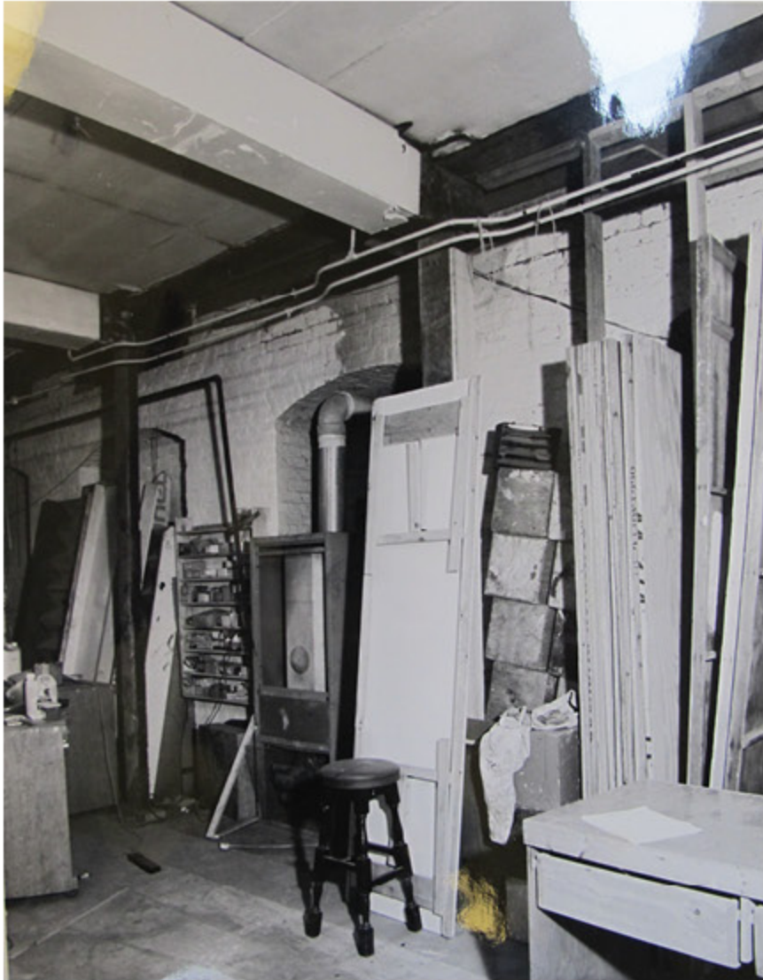
View of the Ground Floor of 28 Macklin Street (circa-1980) showing the exposed timber beams and columns (English Heritage Archive)
