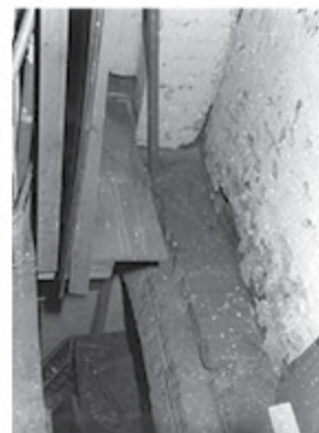
Photograph (28 Macklin St, date unknown) showing the gap between the brick side wall and the floor slab ground floor showing that the paintframe did pass to the basement level. It also shows that at ground floor the gap did not go right into the brick arch (Theatres Trust)
