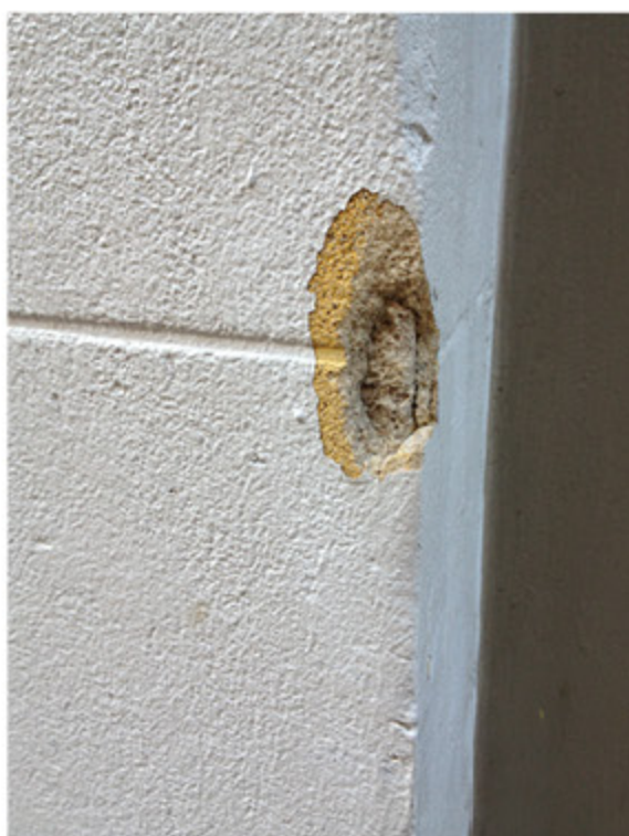
Detailed photograph of facade render (applied in the 1990s) exposing the 15mm thick cement slurry, a fine scratch coat and a more coarse top coat.
