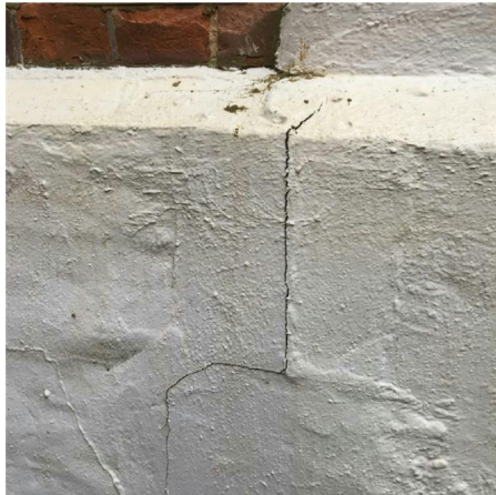
Crack to tight flank wall of the rear projection
