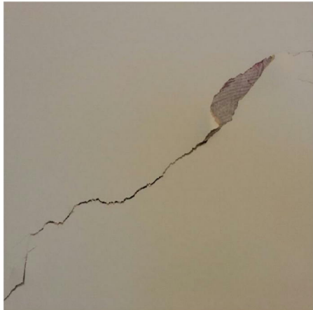
Crack to left flank wall of the meeting room
