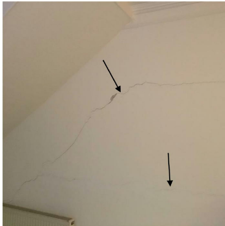
Cracking to the left flank wall of the meeting room
