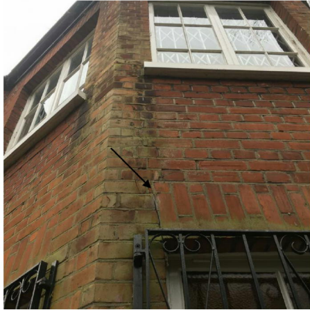
Cracks over the rear bay windows
