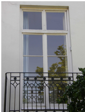
Photo of one of the existing French windows.
