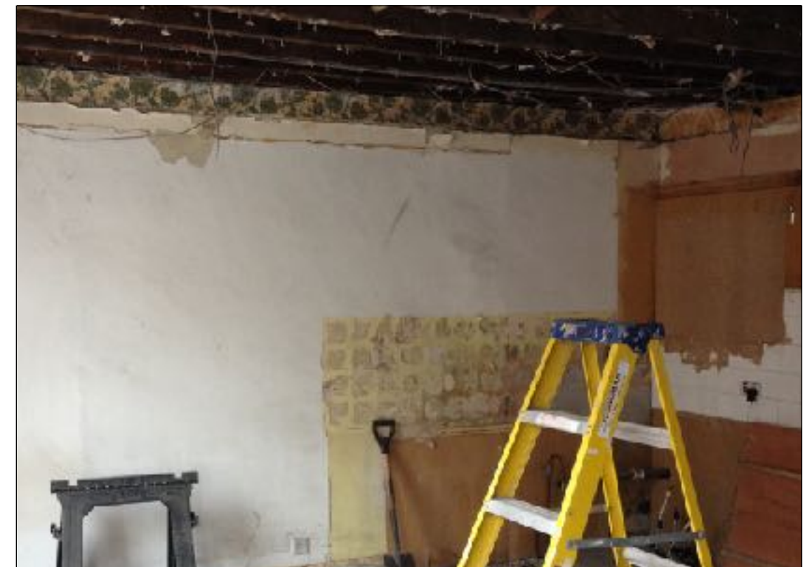
Above and left ; The previous contemporary ceiling was set approximately 300mm below the ceiling joists as evidenced by the early period wallpaper band. The purpose of suspending the ceiling in this manner is unknown.
