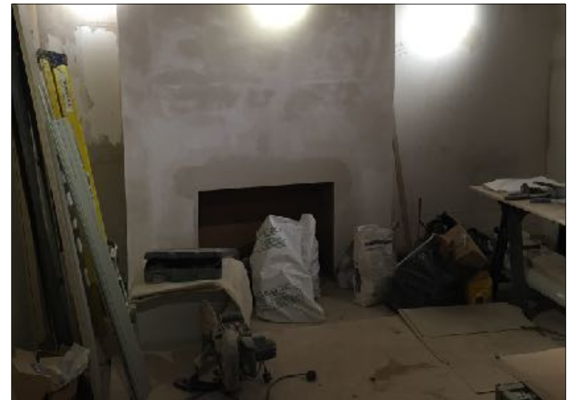
Above : The fireplace aperture post plastering
