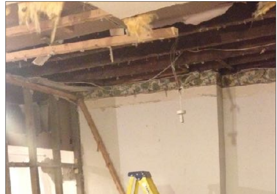
Above : Modern insulation in situ
