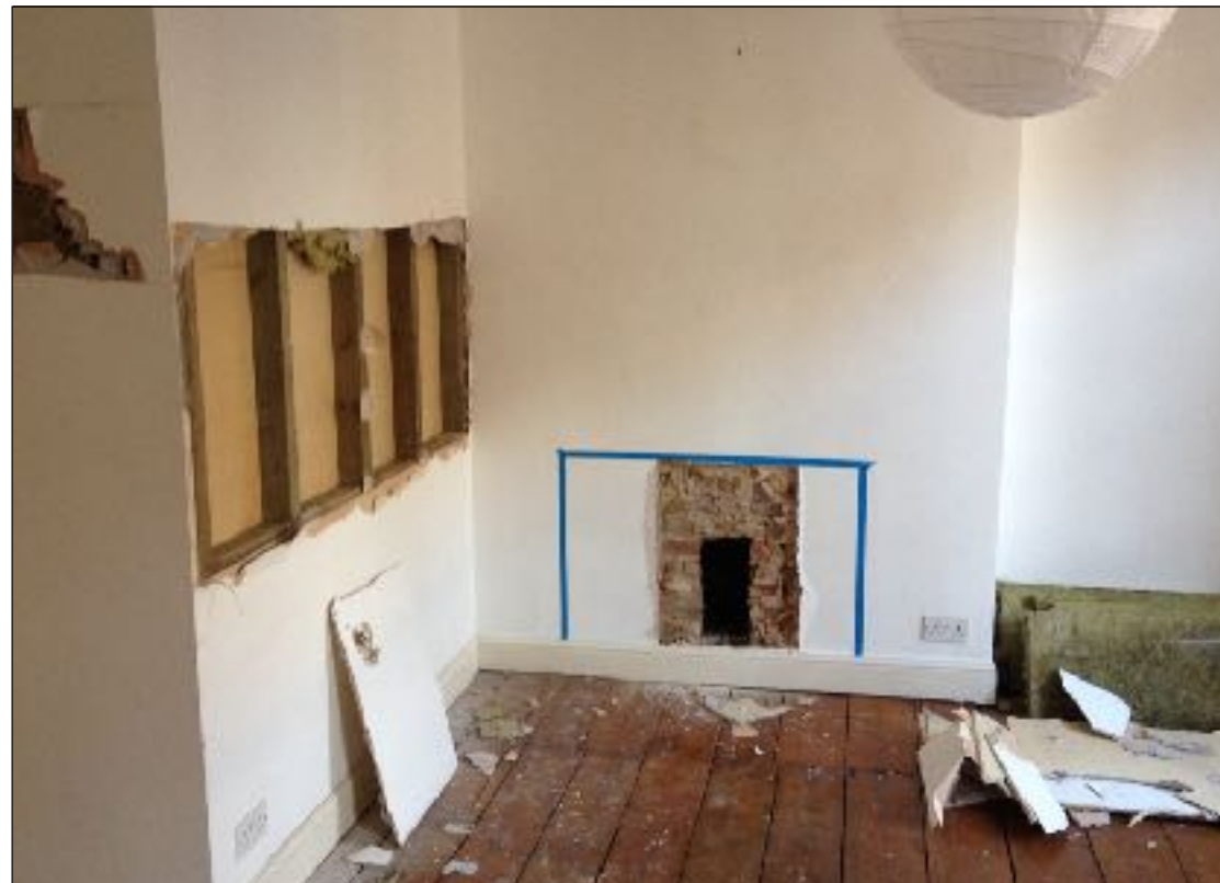
Above and Right : The exploratory aperture made and extent of the fireplace opening marked with blue tape. The rough masonry infill referred to in the text to to the left can be seen above
