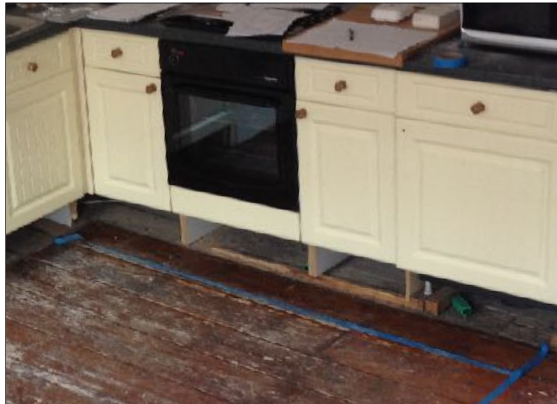
Above : Levelling shims set under the modern kitchen units
