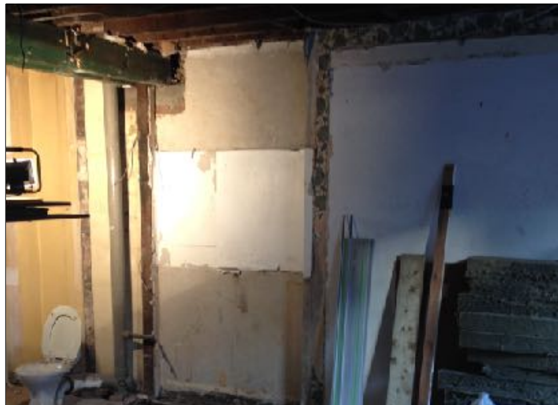
Above and left ; The previous contemporary ceiling was set approximately 300mm below the ceiling joists as evidenced by the early period wallpaper band. The purpose of suspending the ceiling in this manner is unknown.
