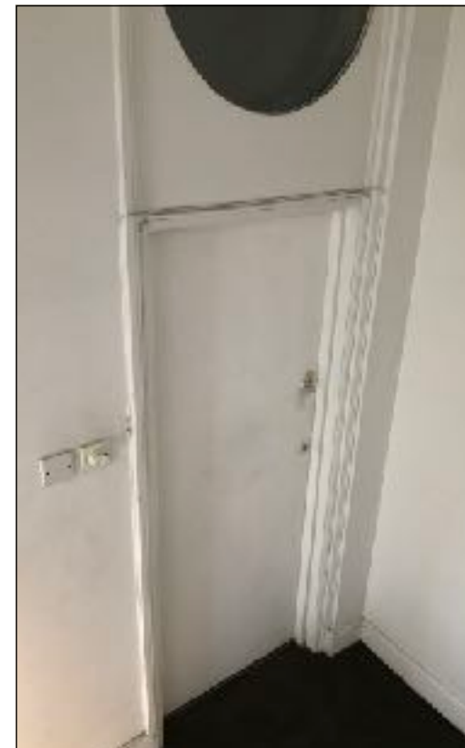
Above: Entrance door to another apartment in the building (Flat B, 1 st floor)
