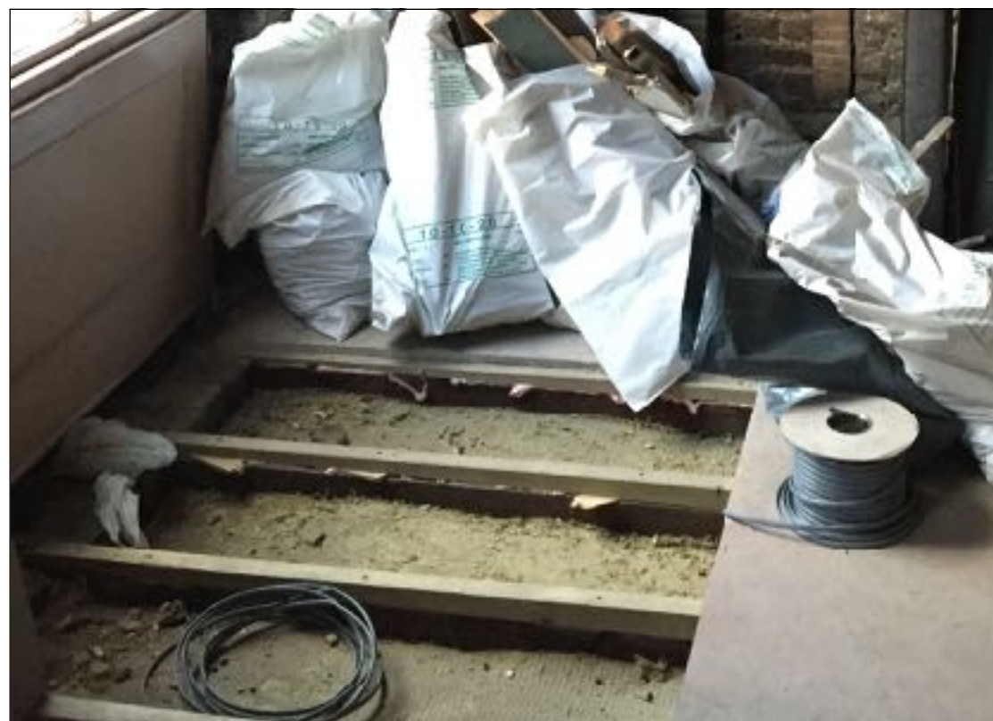
Above : Levelling fillets to support the new floor deck
