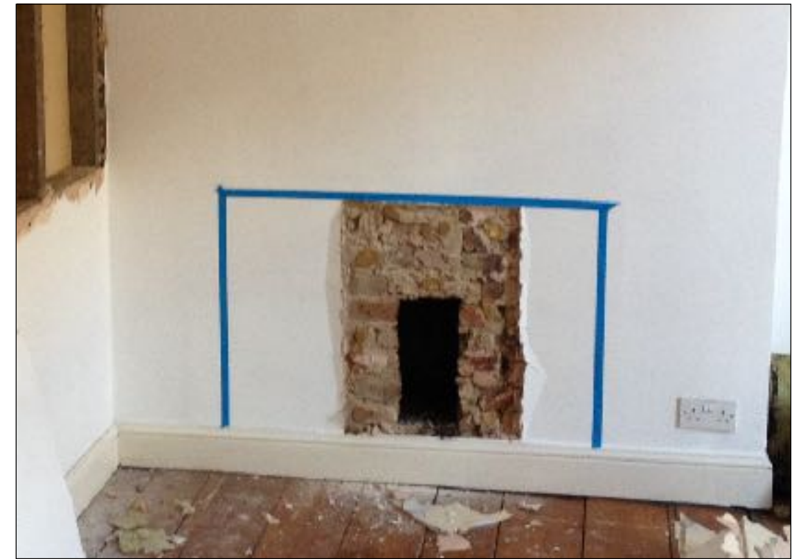
Above : The same skirting pattern was found throughout the apartment possibly indicating complete renewal when the apartment was last refurbished.
