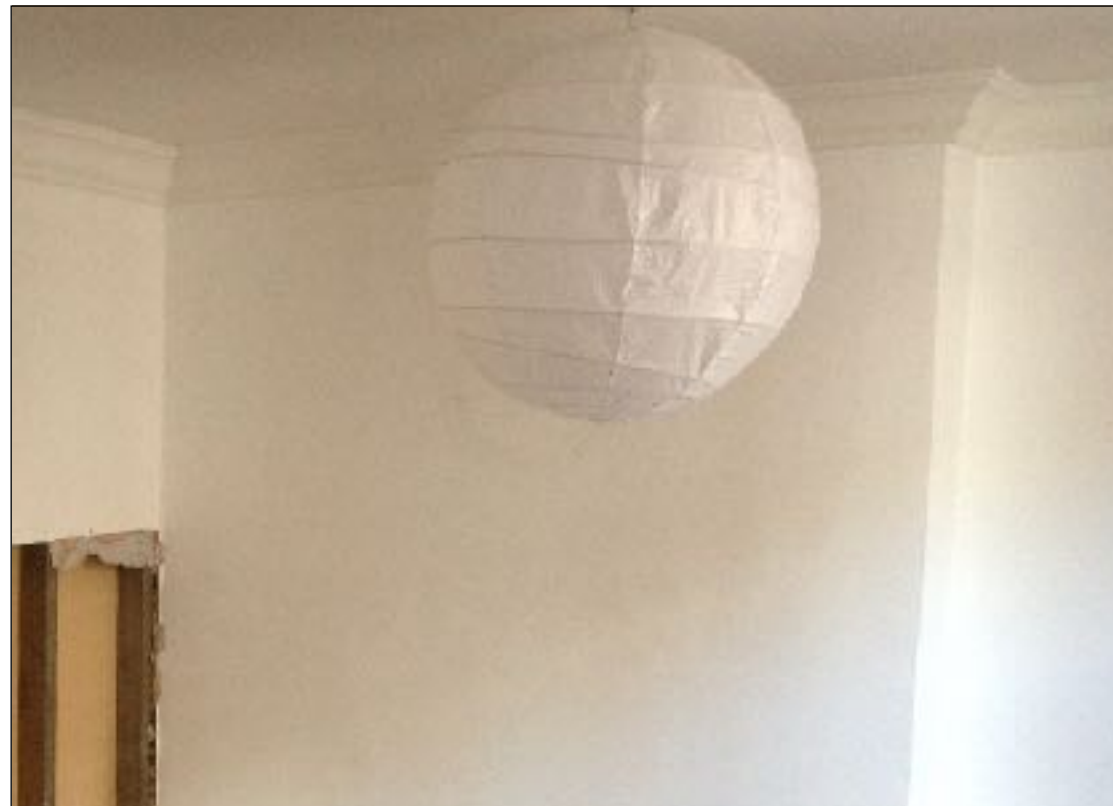
Above : The ceiling and coving prior to renewal works
