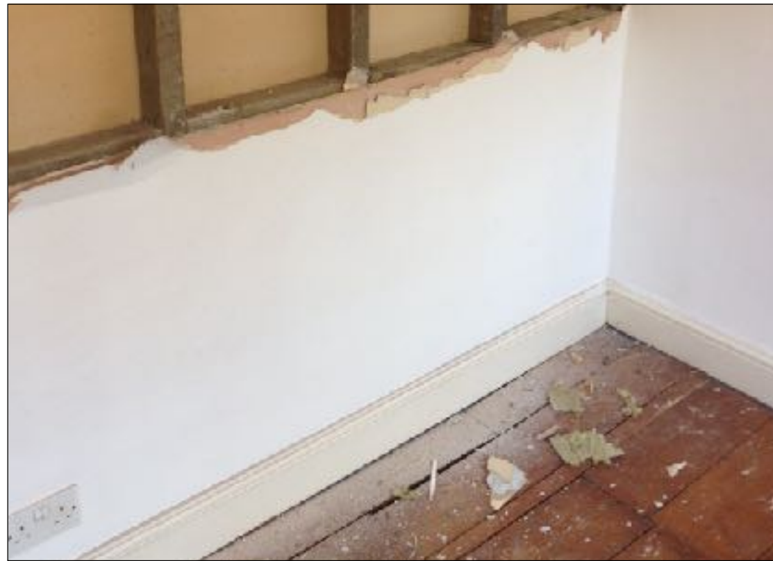
Above : Skirtings to the modern partition wall indicate their placement within the last 25 or so years
