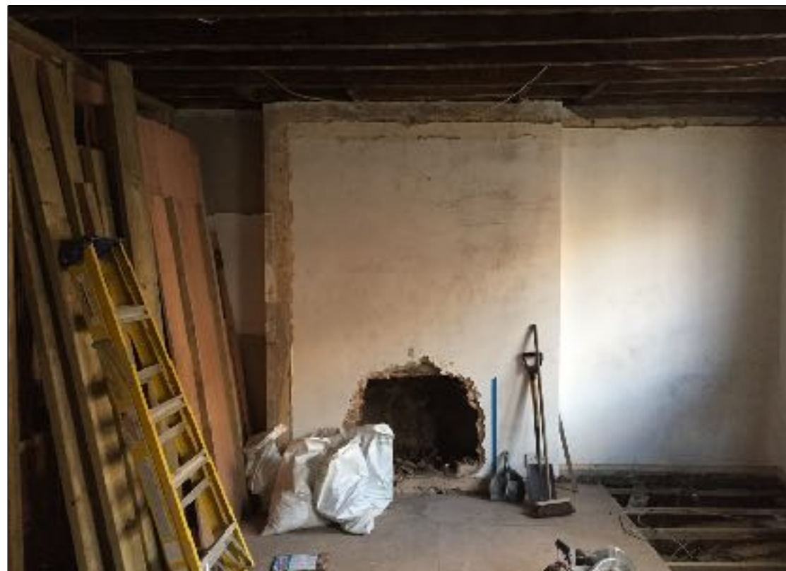
Above : Opening up works in progress
