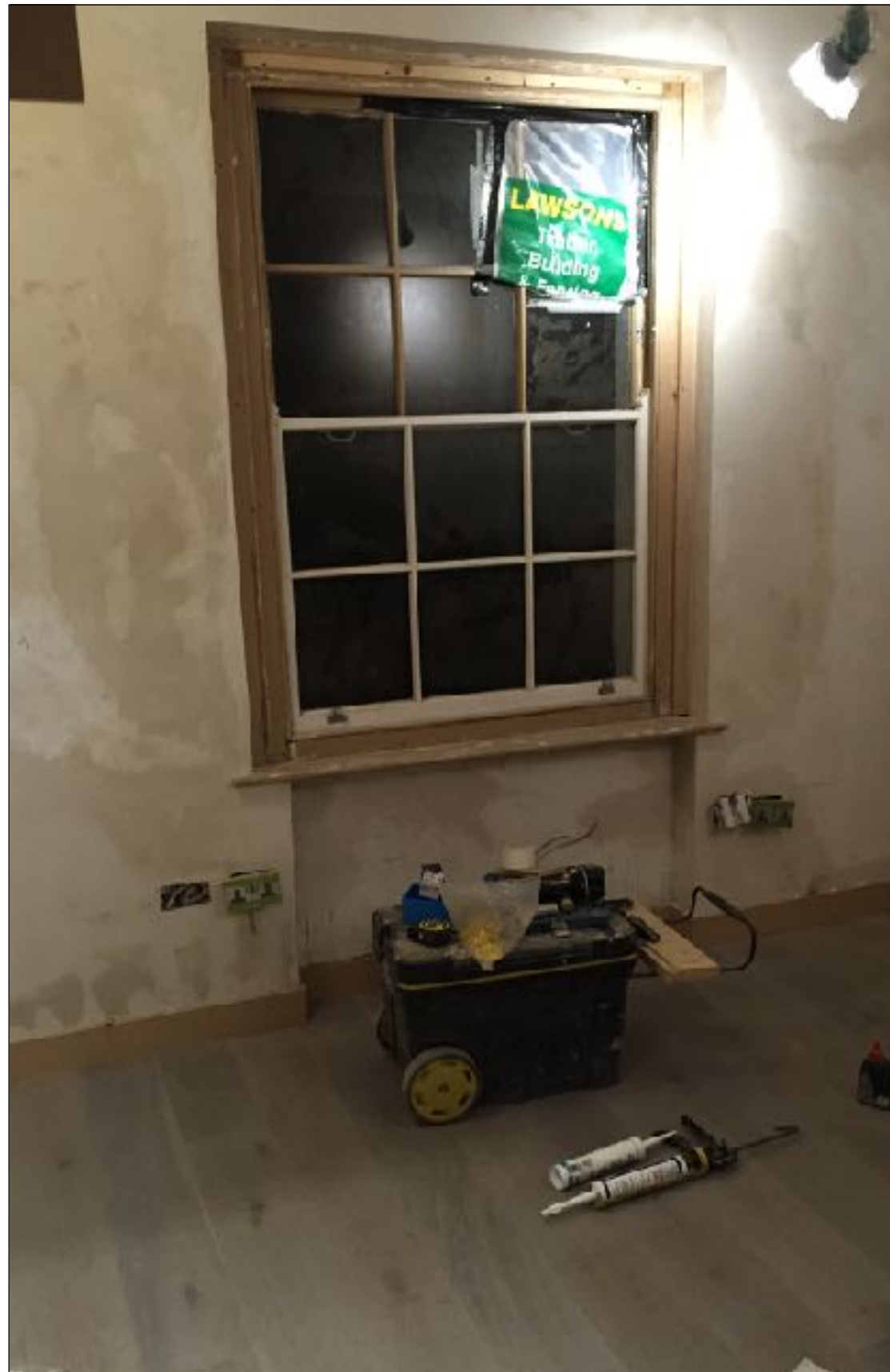
Above : Window to the rear bedroom.
