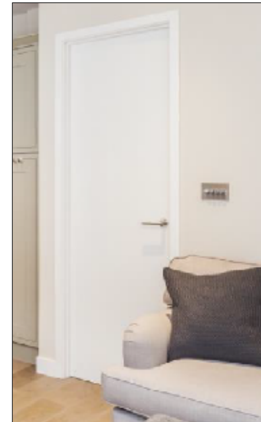
Above : Replacement fire-rated internal door within apartment
