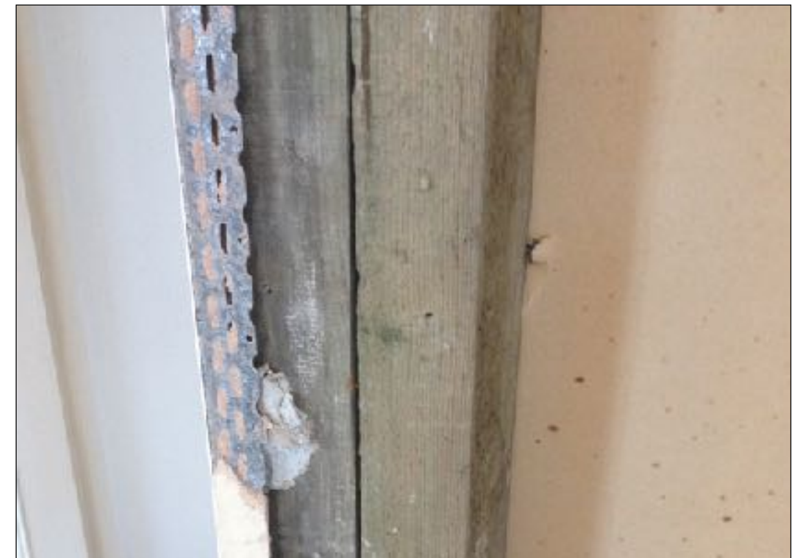
Above : Modern galvanised plasterboard edging within partition
