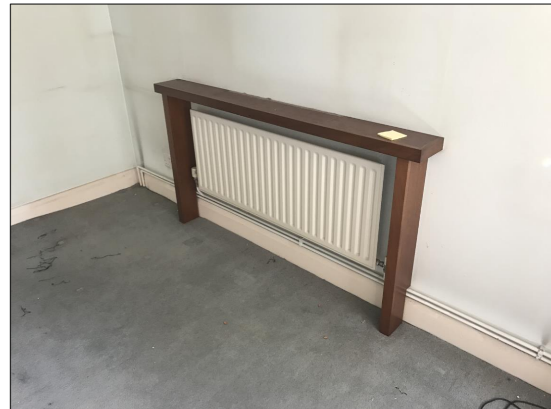
Figure 9 Radiator to be removed. Located in existing third floor living space.
