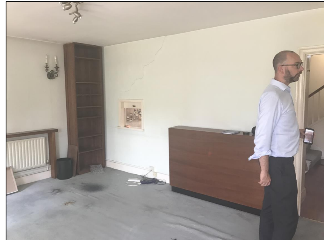
Figure 8 Third floor wall to be removed.
