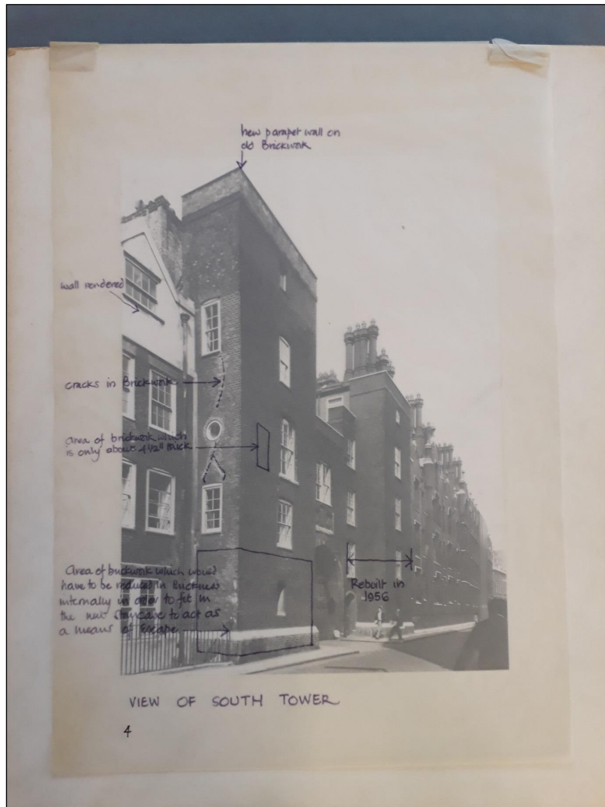
Figure 3 Annotated Photograph of the gatehouse showing the new parapet
