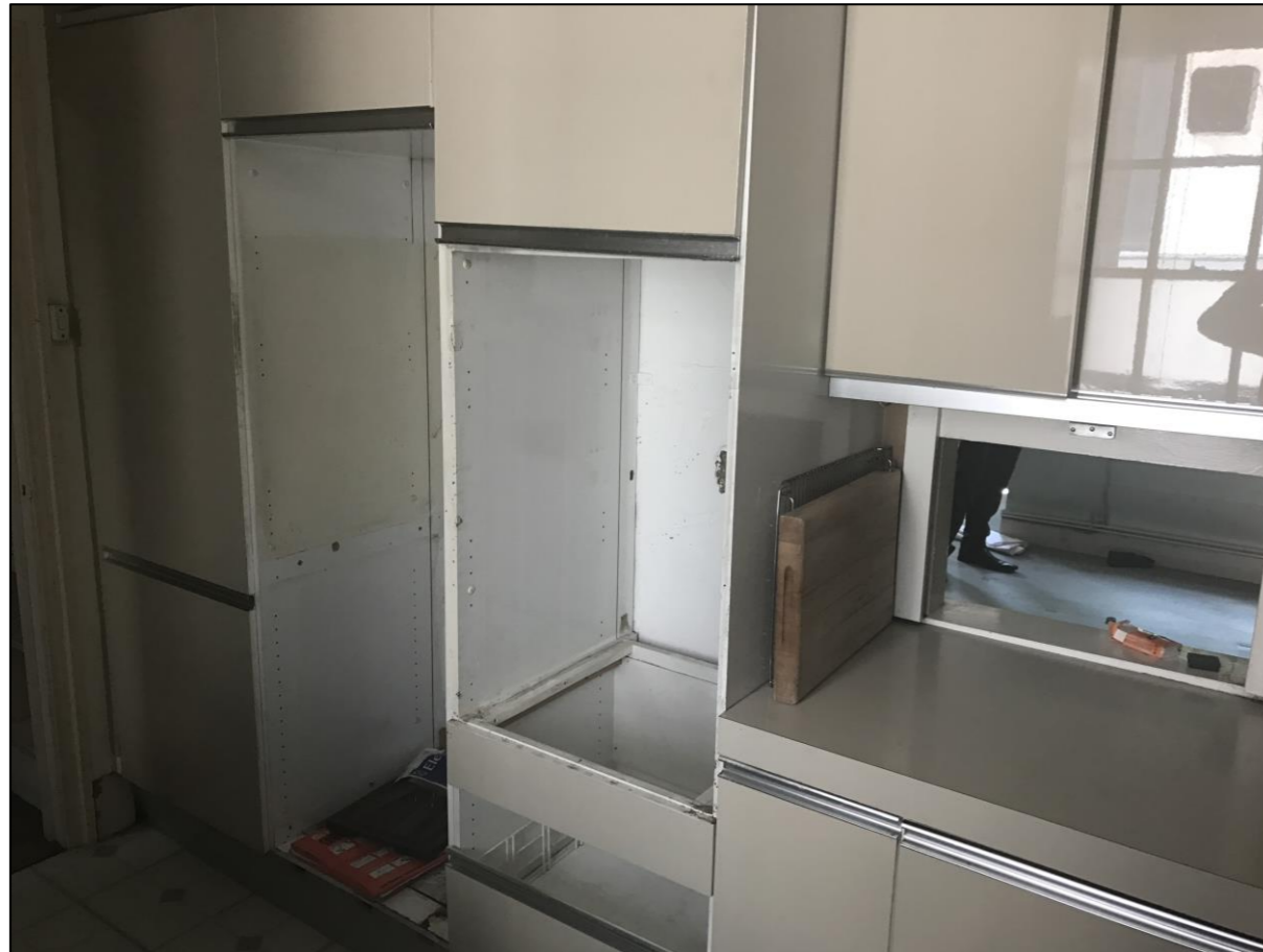
Figure 7 Third floor wall to be removed. Photograph taken from existing kitchen.
