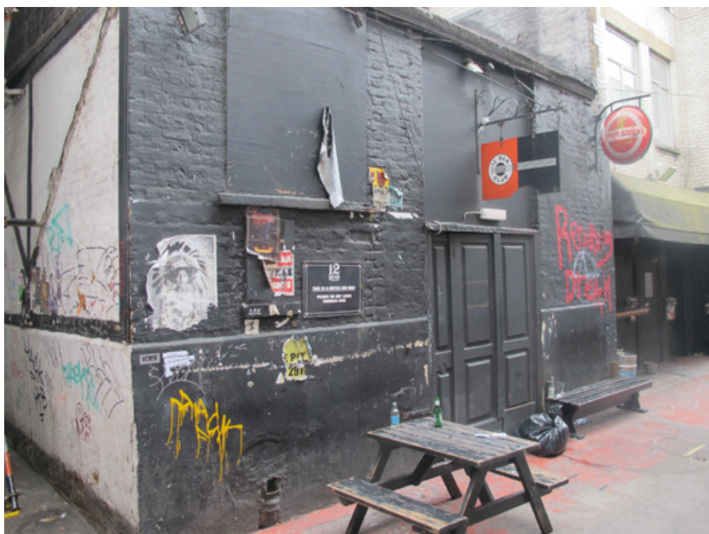
No. 22, the north façade to Denmark Place, showing blocked windows and modern applied timbering (left)
