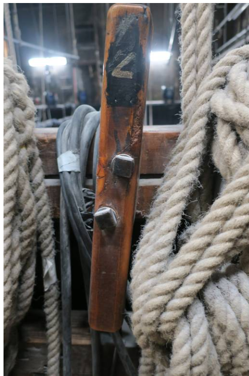
Detail of Timber Fly Rail Cleat (below)
