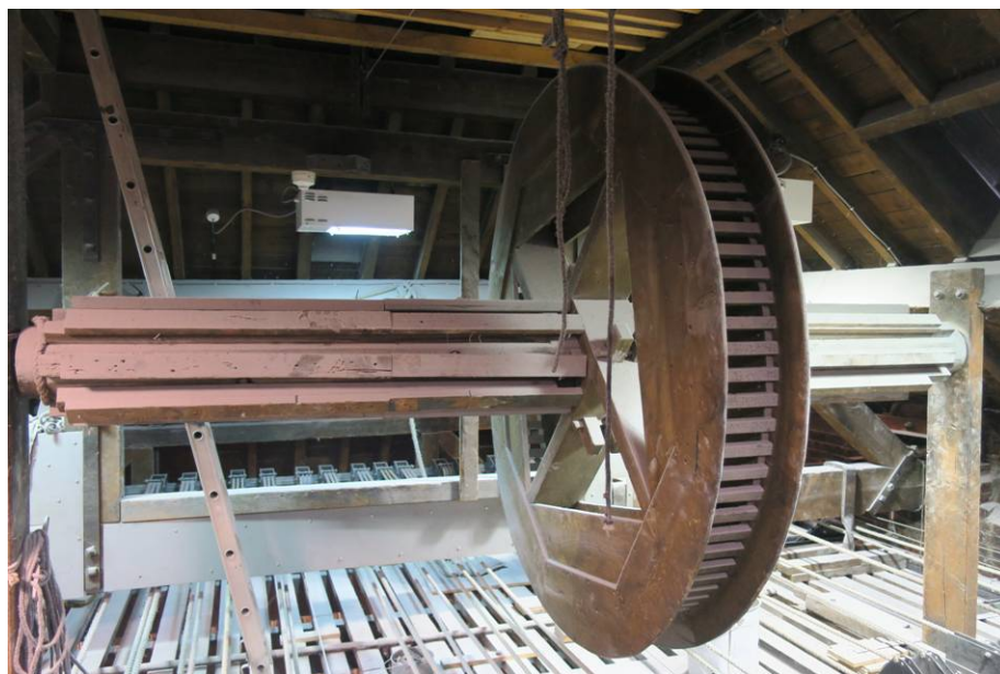
Drum and Shaft at Grid level [photo: theatresearch]
