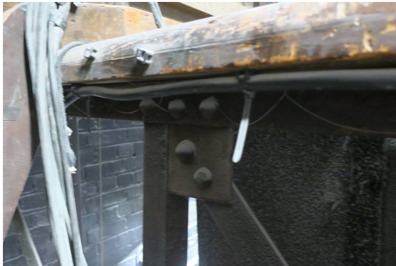
Detail of Fly Rail Construction (above)
