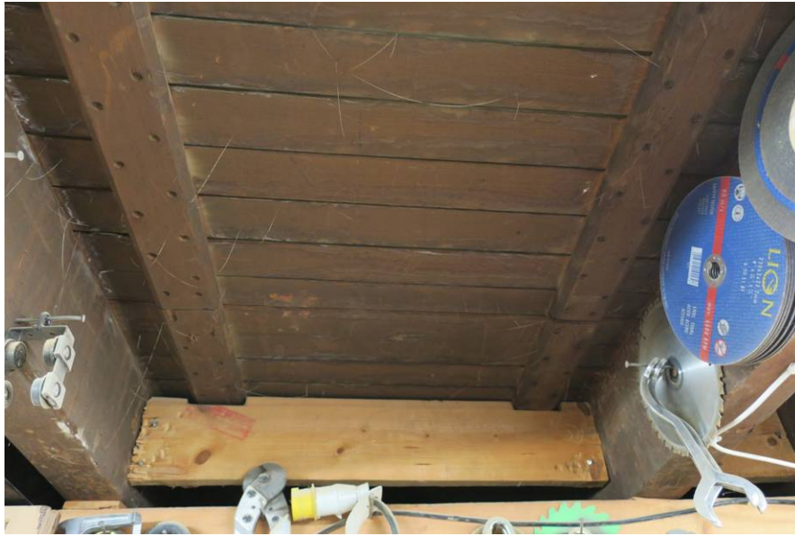
Underside of Scenic Bridge Stage Floor Showing Double Battens [photo: theatre research]
