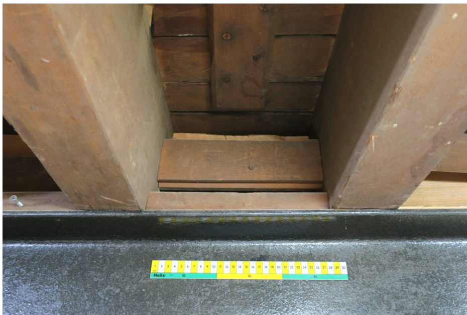
Underside of Stage Floor Single Batten [photo: theatre research]
