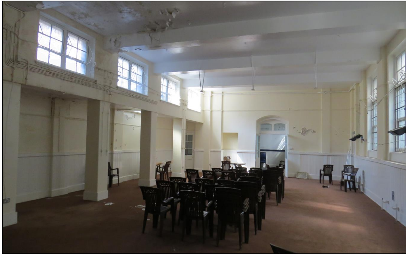
Figure 4.7: The main room in the rear portion of the building at ground floor level.
