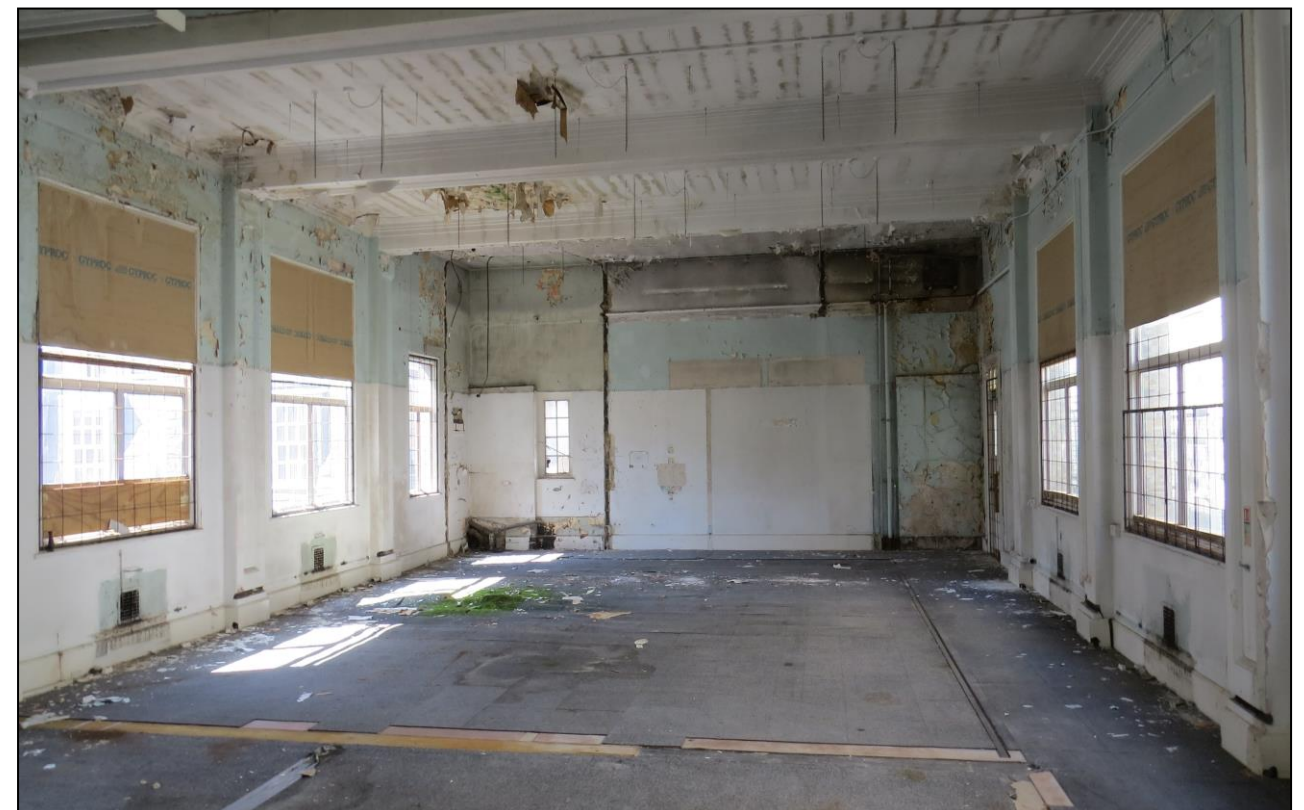
Figure 4.10: The interior of the first floor large room at the rear
