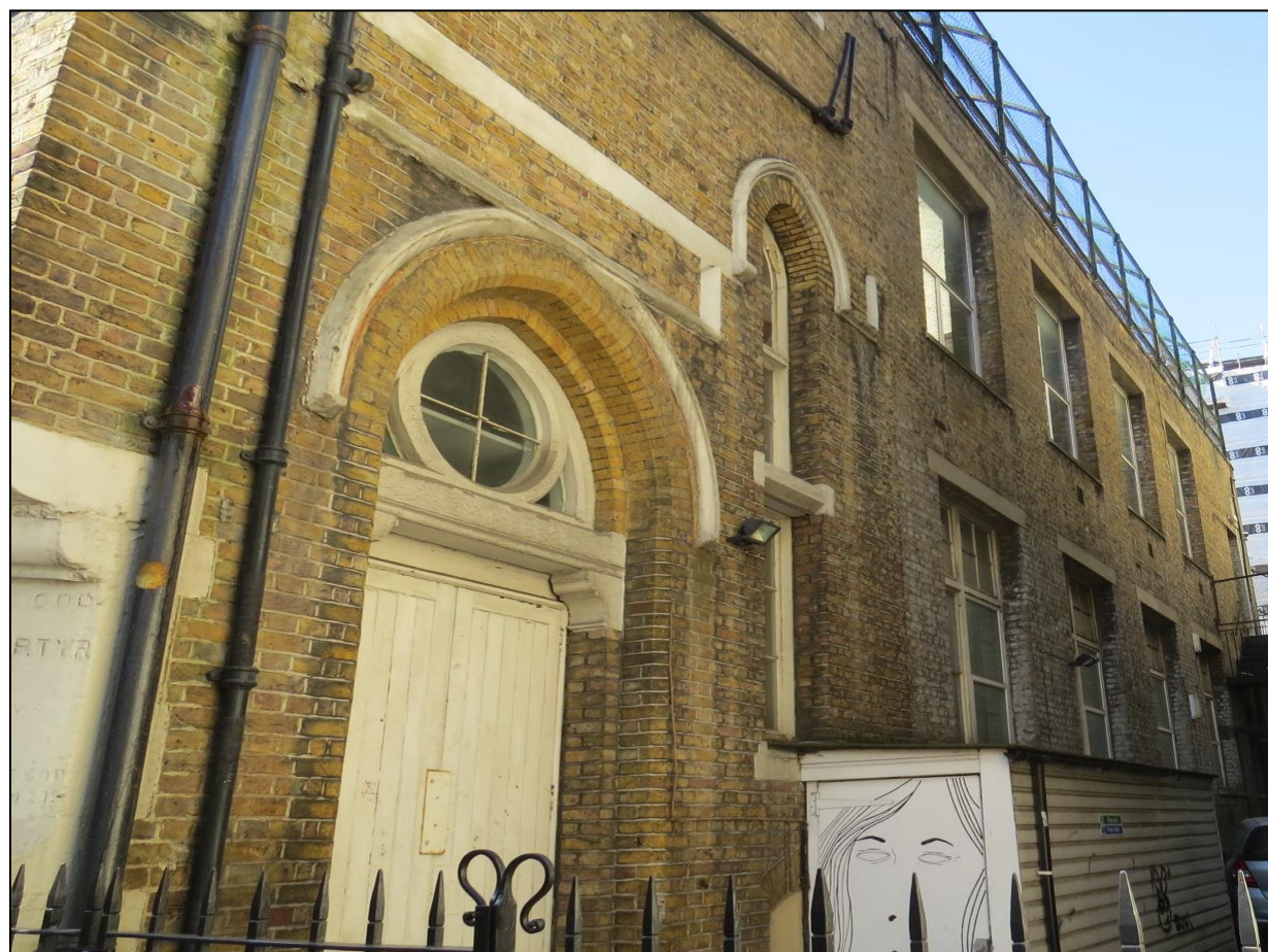
Figure 4.3: view of the north elevation from passageway between the Church and no. 25, with view of window height disparity, change in brickwork, corrugated structure adjacent, and caged structure to rear
