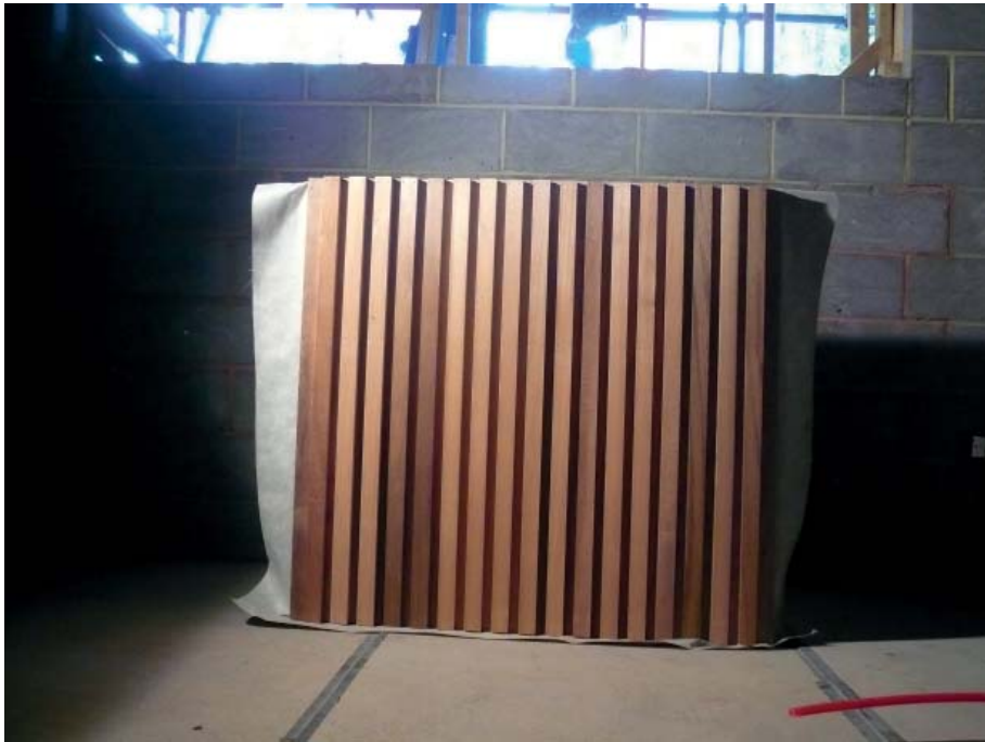
Photograph of sample panel of western red cedar-cladding taken on site.
