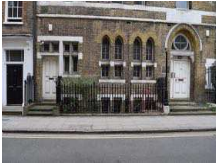
Plate 3- West facing shot of basement entrance from Old Gloucester Street
