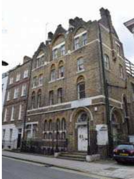
Plate 2- South west facing shot of the exterior of St. George the Martyr School
